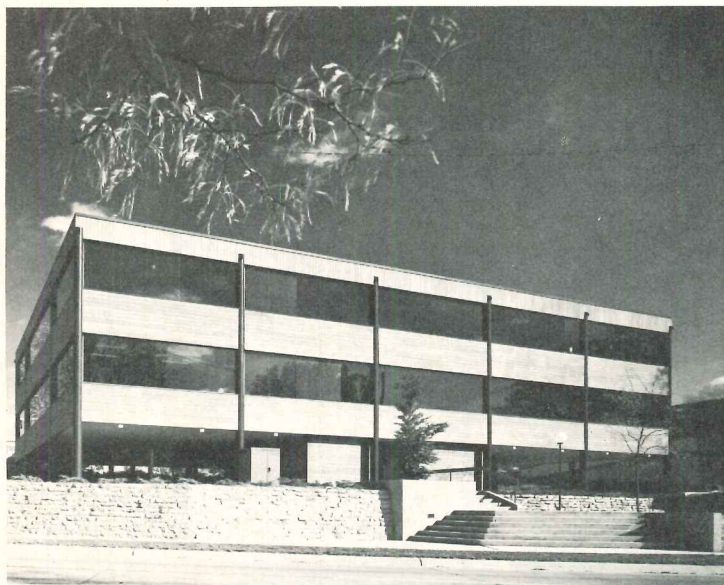
The 101 Southfield building in Birmingham by O'Dell, Hewlett & Luckenbach, Inc. received an award from the Detroit Chapter A.I.A. Other winners were William Kessler & Associates, Inc. for the Bundy Tubing Office Building in Warren; Smith, Hinchman & Grylls, Inc. for the Michigan Electric Power Pool Control Center in Ann Arbor; Eberle M. Smith Associates, Inc. for the Frank Murphy Hall of Justice, Detroit; and Ziegelman & Ziegelman for a Troy bank.
