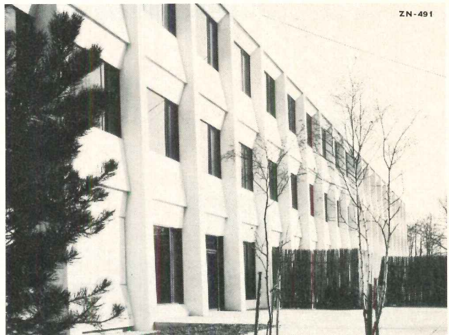
IBM's beautiful Data Processing headquarters utilizes galvanized re-rod to prevent sub-surface rust and consequent staining.
