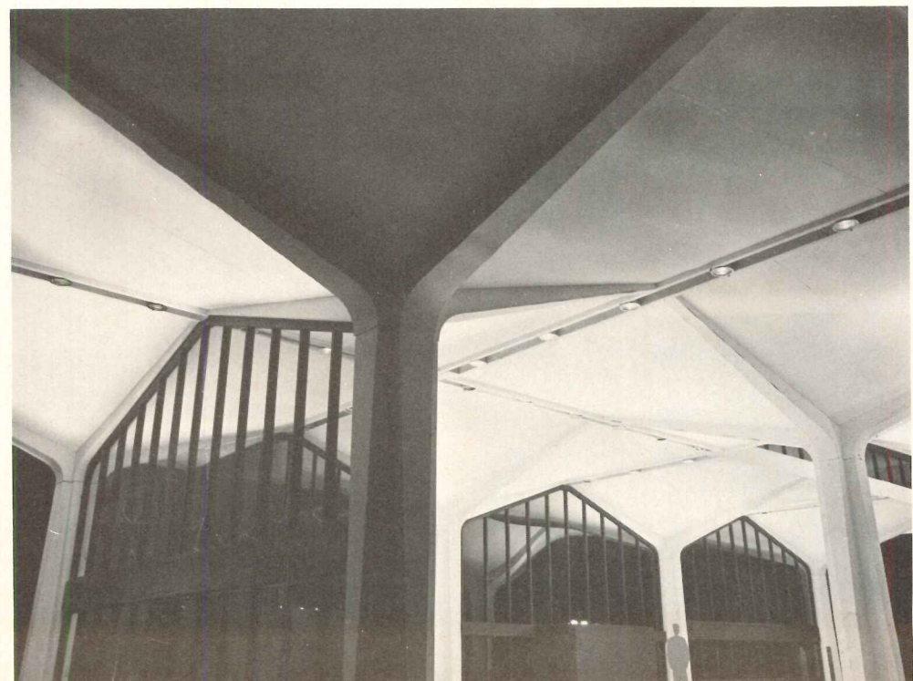
Both uplights and downlights are on in the photo above. Idea was to have maximum brightness at columns and feather out to edge of the umbrellas. Below is photo showing interior and exterior lighting.
