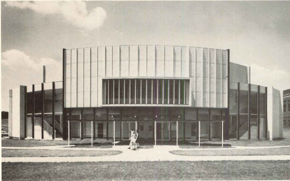
Theater and Classroom Building, Birmingham-Southern College, Birmingham, Ala. Architects: Warren, Knight & Davis. Theater Consultant: Dr. Arnold Powell. General Contractor: Brice Building Company, Inc. Dover Stage Lift installed by Dover Elevator Co., Birmingham.
