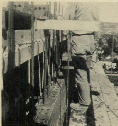
This 14-story housing project turned to brick bearing walls in place of load-bearing precast panels to save on costs while providing an attractive facade. The bearing walls were reinforced from 11th through 14th stories to give added strength for wind loads. Floors were shored to allow concrete work to proceed ahead of brick, and reshored to keep load off brick walls while mortar cured.
