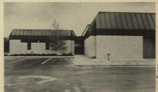
A labor union clinic Architect: Bernard A. Marson
