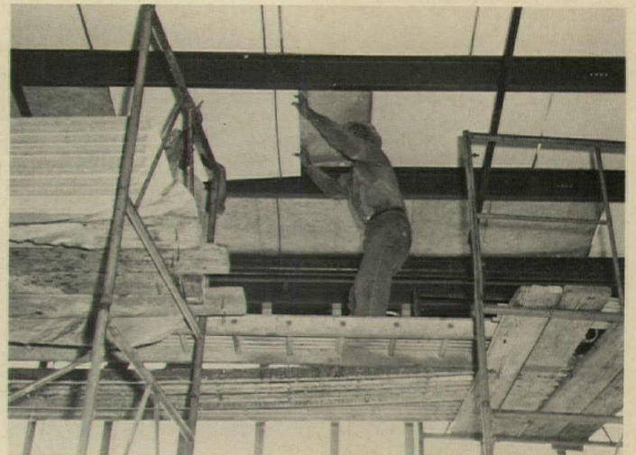
Interior finish frequently used with the system is a heavy-density insulation board painted on one side for appearance and easy maintenance.
