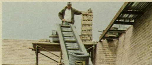
Keywall Multibond comes in rolls that are easy to hand carry, roll, convey, or wheel. One roll reinforces 200 ft.
