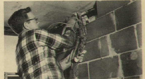
The two components of urethane foam insulation are introduced into the cavity of the exterior wall through hoses attached to a nozzle.
