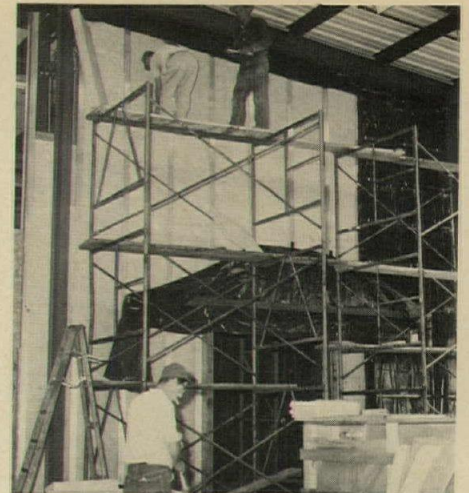
Semi-rigid batts of fiberglass fit neatly between the flanges of the insulated studs.
