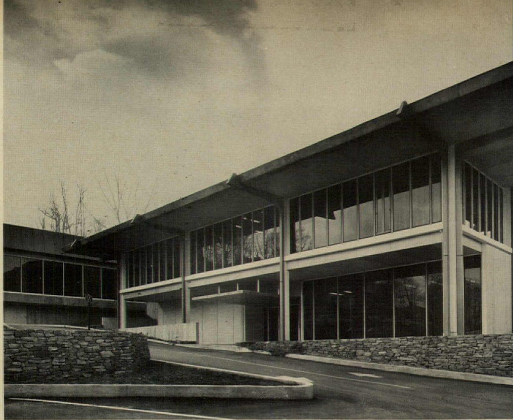
The attic created by the hip roof is used for air conditioning equipment and elevator machinery. Overhanging sides of the roof reduce solar heat gain.
