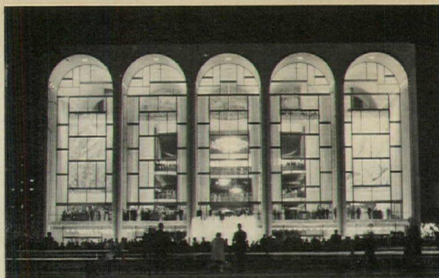
METROPOLITAN OPERA, Lincoln Center, New York City — Seven 8' x 60' stage lifts, two orchestra pit lifts, other equipment for handling sets and scenery.
