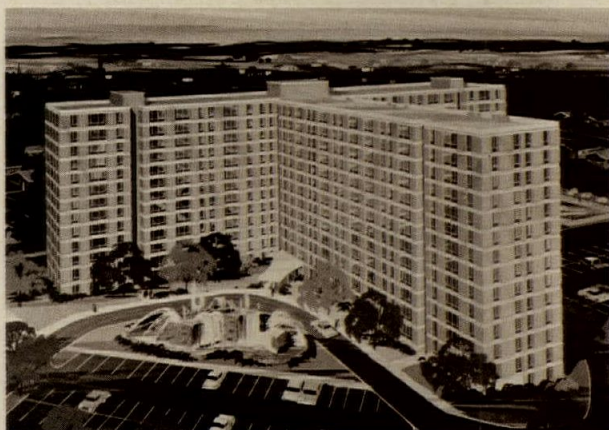
Use of rigid urethane foam as structural insulant for $8-million apartment complex reduced construction costs, could shave $2000 a year from heating and cooling bills.
