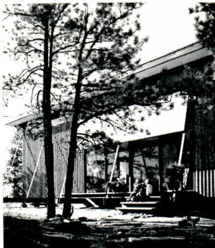
Sun protection is vital for efficient air conditioning, by overhangs or such adjustable
