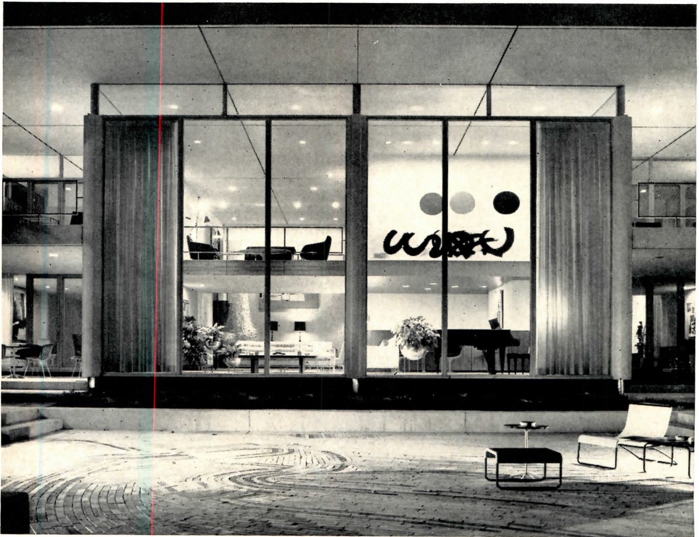
Huge 59" x 189" Therm-O-Proof insulating glass units in Grosse Pointe Shores, Mich. "Record House." Architects: Meathe, Kessler & Associates, Grosse Pointe, Michigan
