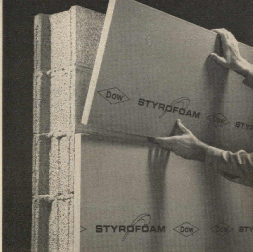
4. Press Styrofoam FR into place. It installs fast, stays dry for year-round comfort.
