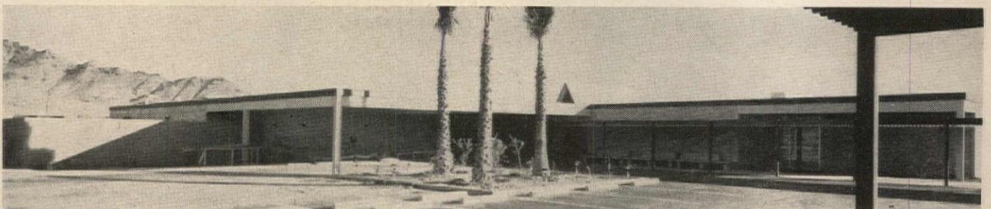
Orangewood, Phoenix, Ariz. Architects: Allan & Olsson, A.I.A. Owner: American Baptist Estates, Inc. Contractor: The Edward Gray Corp.
