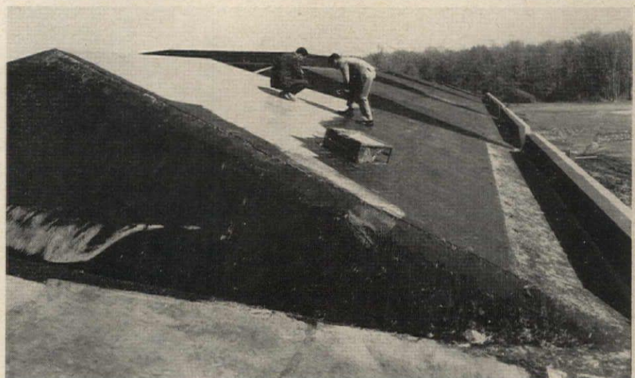
Above: Fluid roofing can be reinforced with chopped glass fibers blown on the wet neoprene film. Below: Light colored top film of Hypalon has been partly finished
