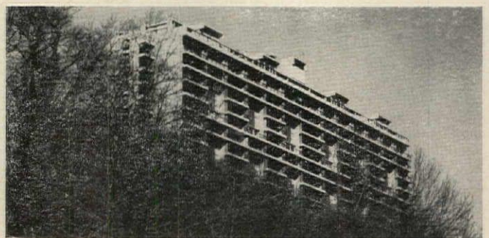
FIRST HONOR AWARD: Horizon House, Fort Lee, New Jersey. ARCHITECTS: Kelly & Gruzen; LANDSCAPE ARCHITECT: Michael Burris; BUILDER: Tishman Realty & Construction Company. Structural system on a 24-foot module utilizes 8-inch concrete bearing walls and 8-inch flat slabs to provide clean, unbroken walls and ceilings throughout. The jury: "Imaginative use of concrete as exterior finish—direct, handsome."
