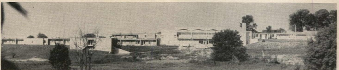
Pilgrim Manor Home for Senior Citizens, Grand Rapids, Mich. Architects: Wold & Bowers, Architects Owner: Pilgrim Manor, Inc. Contractor: George Datema & Sons
