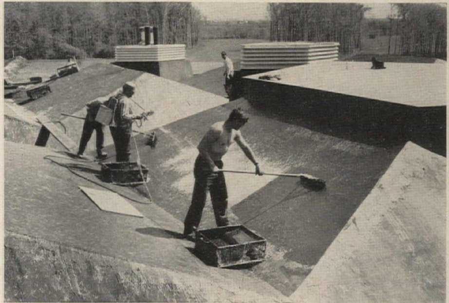
Above: Fluid roofing can be reinforced with chopped glass fibers blown on the wet neoprene film. Below: Light colored top film of Hypalon has been partly finished
