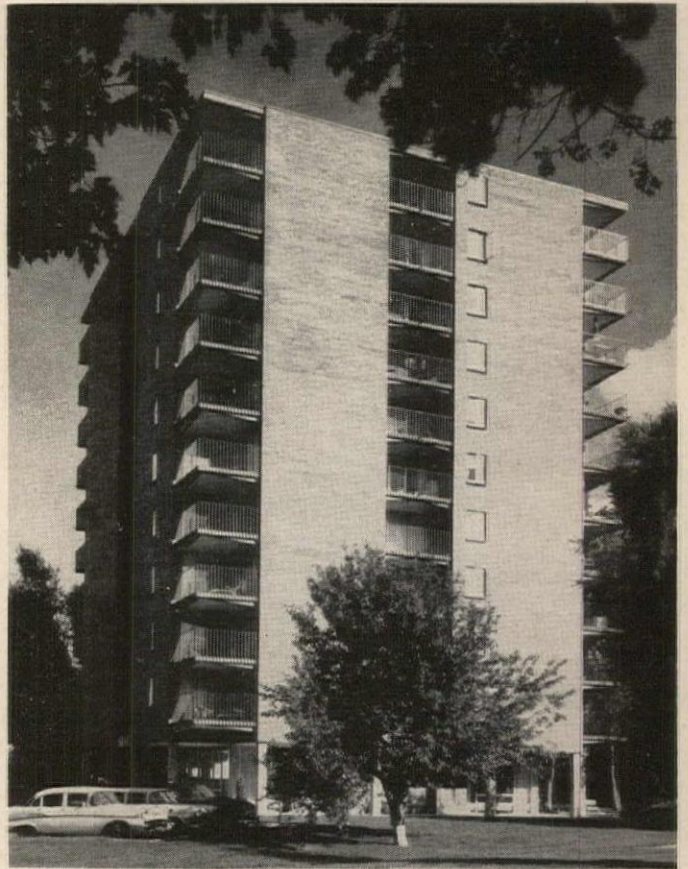
Presbyterian Manor, Boulder, Colo. Architect: Hobart D. Wagener Owner: Boulder Presbyterian Housing, Inc. Contractor: Brown Schrepferman & Co.
