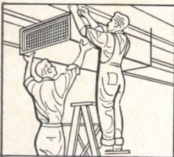
Central-Air Unit ceiling mounts in basement; supplies base heat load, cooling, electrostatic filtering, humidification and deodorizing.
