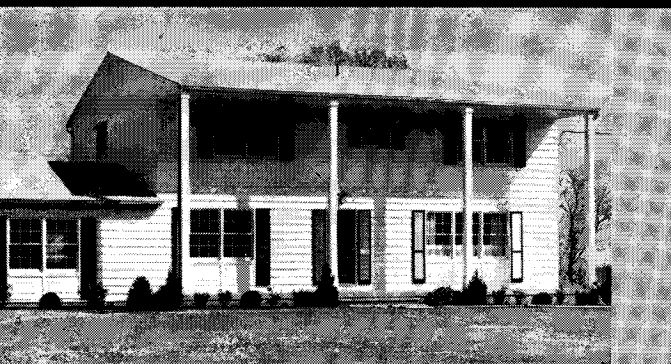
THIS IS FIRST OF 172 hydronic homes to be erected on \frac{1}{2} acre plots in New City, Rockland County, New York.
