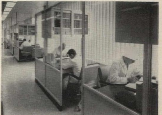
Desk space for chemists and technicians is in the same room as work benches, but is separated from the room by partial-height glass partitions which serve also as splash shields. Over the desks are enclosed bookcases. Each desk has a lab-type electrical outlet for plugging in such equipment as microscopes or business machines. Vertical blinds control daylight
