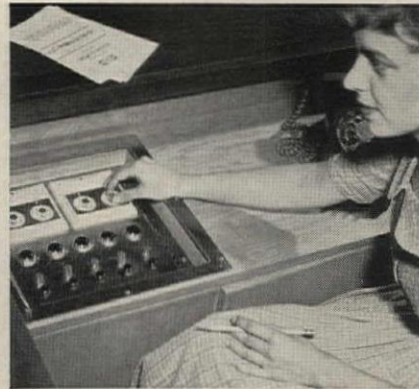
Receptionist has fingertip control of regular and emergency lights with G-E Selector Switches built into desk.
