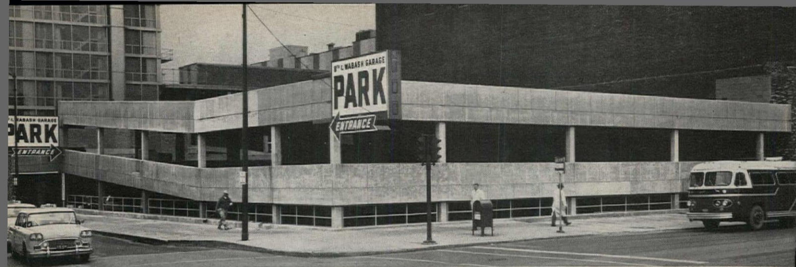
8th and Wabash Corporation Parking Garage, Chicago. Designed by Miller Engineering Company; built by Stuparitz Construction Company; both of Chicago. Area: 65,000 sq. ft.
