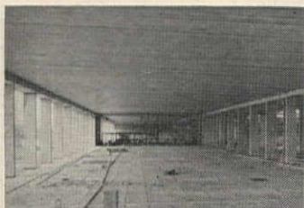
Long span Hi-Stress ceiling before partitions installed.
