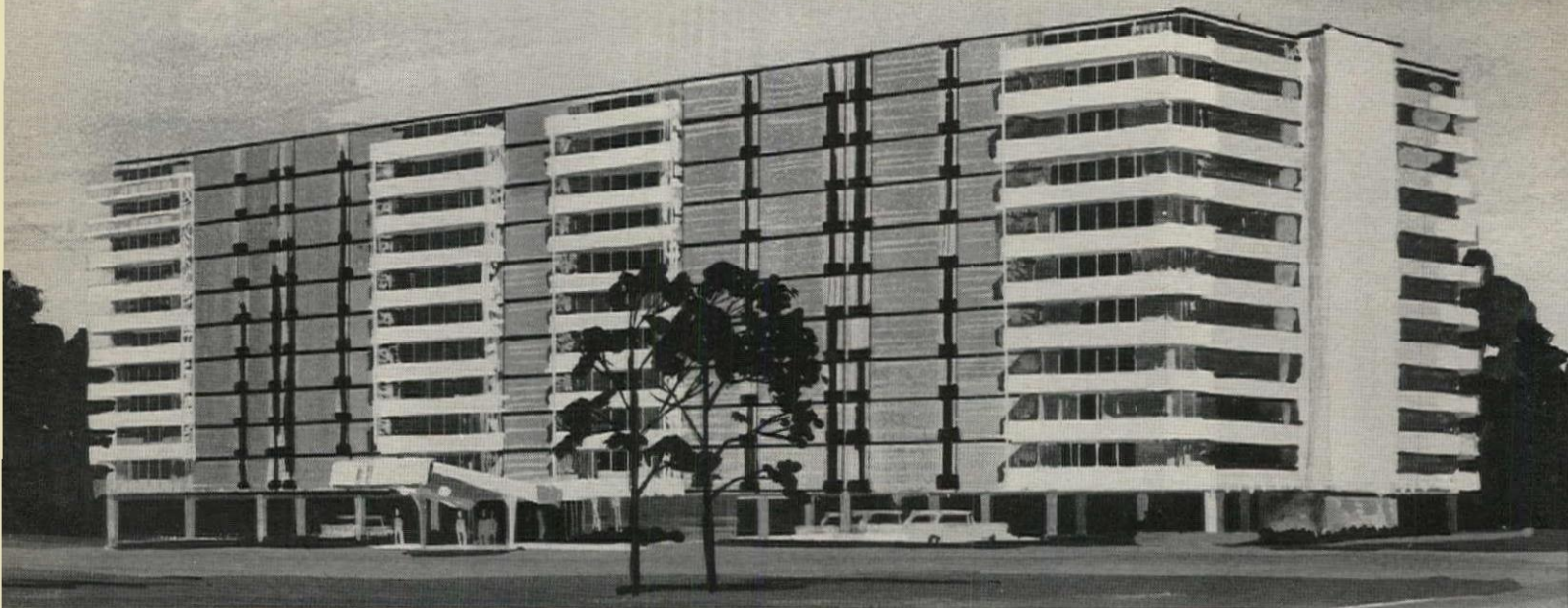
Owner-Builder: BCH Construction Corporation; architect-engineer: Backus, Crane & Love; steelwork: Bethlehem Steel Company.
