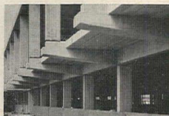
Lateral beams at second floor cantilever 7'-3".
