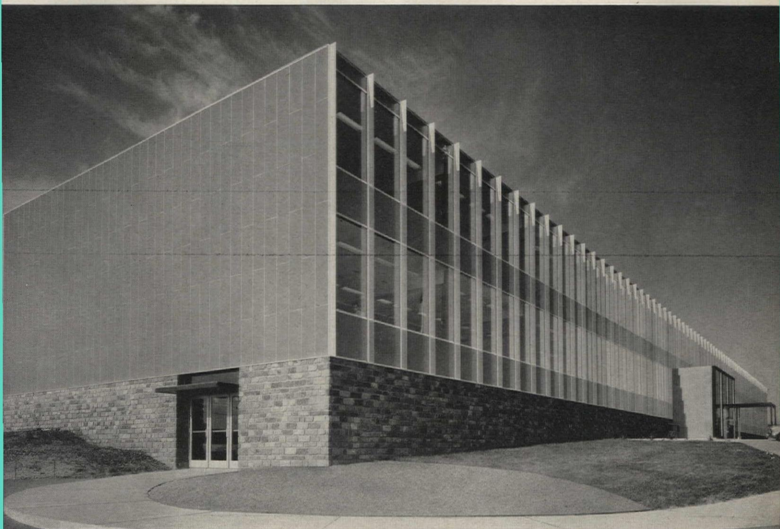
McDonnell Aircraft Corporation Engineering Campus at St. Louis, Mo. Architect: Harris Armstrong, F.A.I.A. Panels made by Atlas Enameling Company, Inc., St. Louis. General contractor, Gamble Construction Company, St. Louis.
