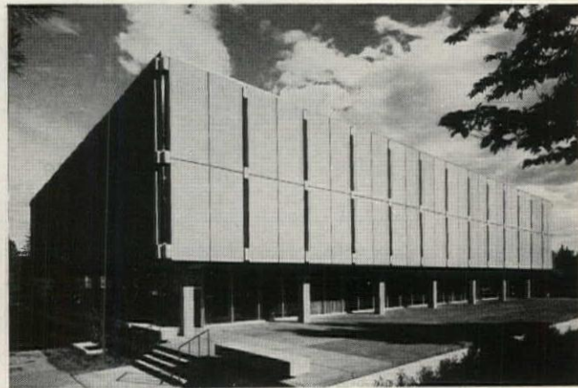
Tutt Library, Colorado College, Colorado Springs. Architects: Skidmore, Owings & Merrill. Contractor: Lembke Construction Company of Colorado, Inc. Rotary Oilraulic Passenger Elevator sold and installed by Dover Elevator Co.
