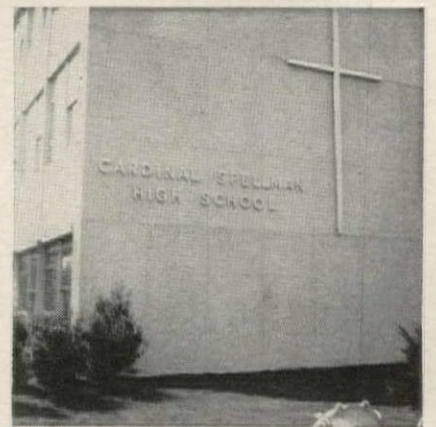
Cardinal Spellman High School Bronx, New York Architects: Eggers and Higgins Installation by: Abbott-Redmont Thinlite Corp., New York, New York
