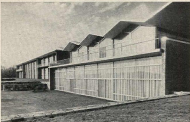
New Raytheon Executive Offices, completed in 1961. Architects: Anderson, Beckwith, and Haible; General Contractor: George A. Fuller Company; Consulting Electrical Engineer: Edwin Mahard; Electrical Contractor: M. B. Foster Company. (All of Boston.)
