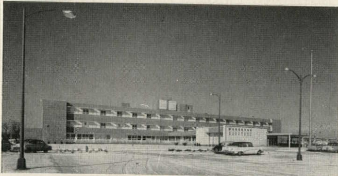
MCDONOUGH HOSPITAL, MACOMB, ILL. TROY-PLANNED LAUNDRY FOR ARCHITECT LANKTON-ZIEGELE-TERRY AND ASSOCIATES, PEORIA, ILL.
