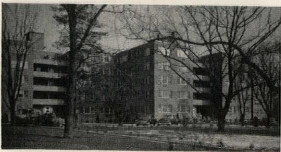
Trouble-free Donley Incinerators were specified for this large residential development in Philadelphia.
