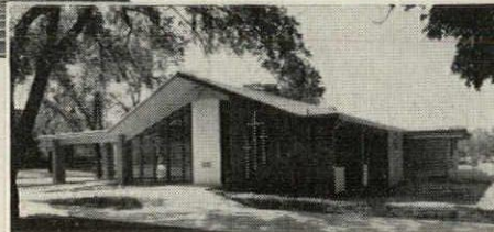
■ St. Joseph's Catholic Church — Yates Center, Kan., 21 Rilco beams varying in length from 4'2" to 39'.
