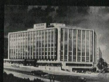
Universal Building, Washington, D. C.; LeRoy Werner, Architect
