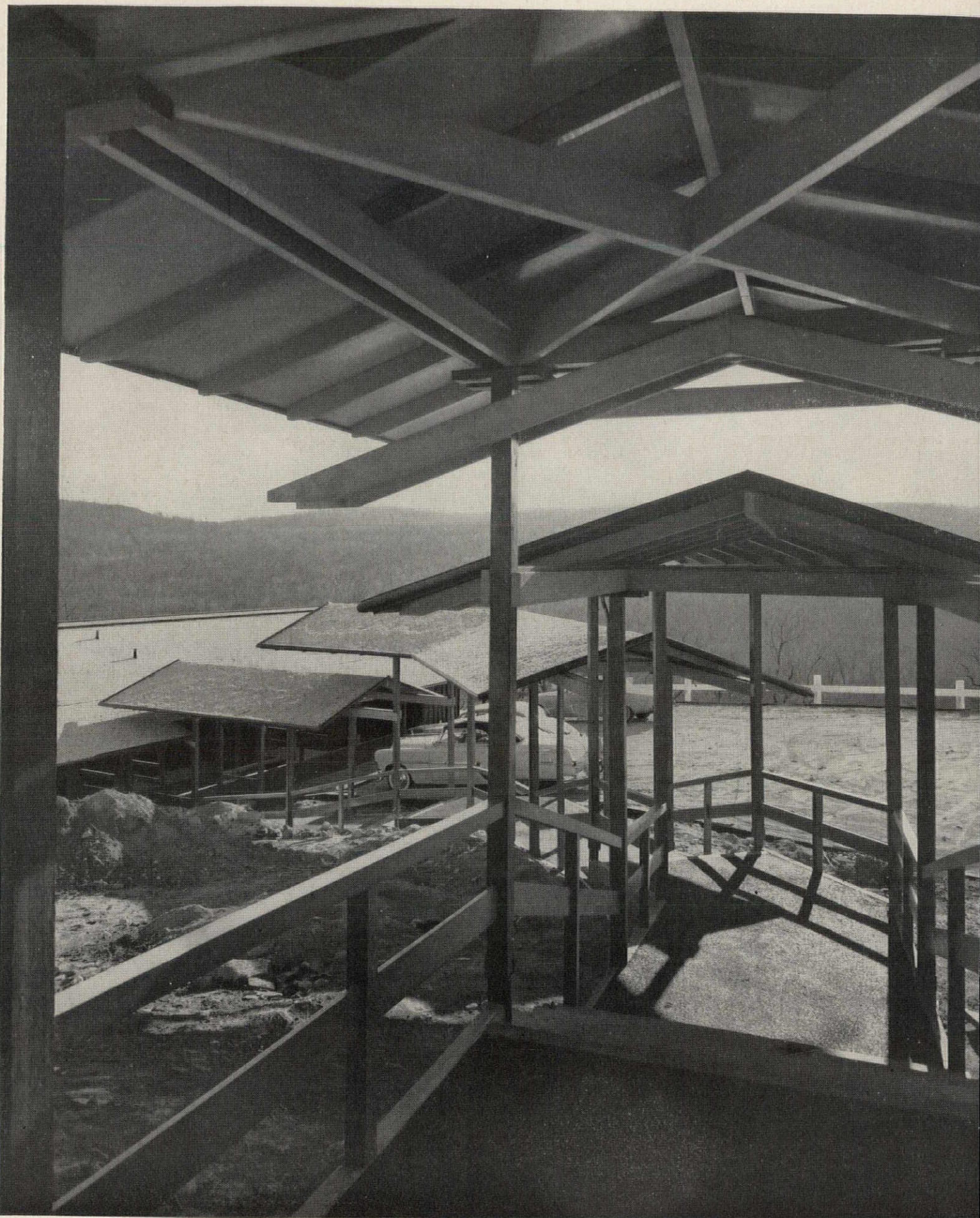
Chosen for its workability and ability to blend with the beauty of the landscape, straight grain wood is utilized in exposed framing throughout the Motel on the Mountain, Suffern, N.Y. Architects: Harwell Hamilton Harris, Perkins and Will.
