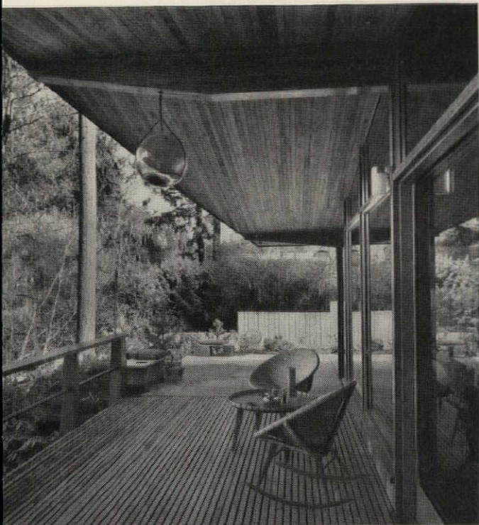
Exposed framing, 2" lumber on edge in decking and ceiling, on the porch of this new Lake Grove, Ore. lakefront home, form a natural setting for a scenic view. Architect: Van Evera Bailey.
