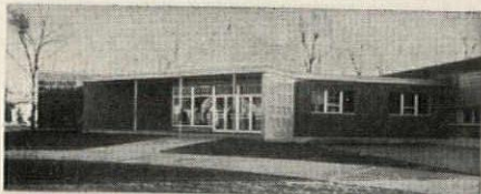
Midway Manor Elementary School - Allentown Arch.: Heyl-Bond-Miller, Allentown
