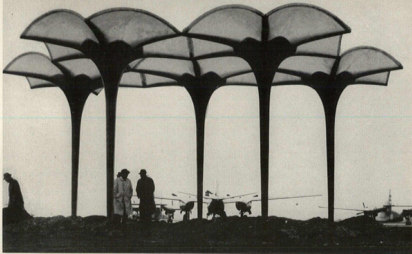
Five-parasol cluster set up at the intersection of two runways at Long Island's Mitchel Air Force Base was tested for dynamic behavior under made-to-order gales provided by the slipstreams from the props of the two B-26's shown in the background
