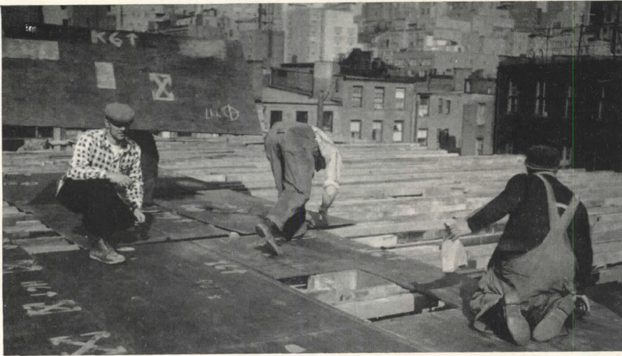
After setting up column forms and framing for decking, workmen lay plywood deck forms for flat plate slabs. Markings indicate the position of each panel, as well as the location of each break in the slab. Three sets of forms, all identically marked, were used on the job, requiring only verification of markings as each floor was formed
