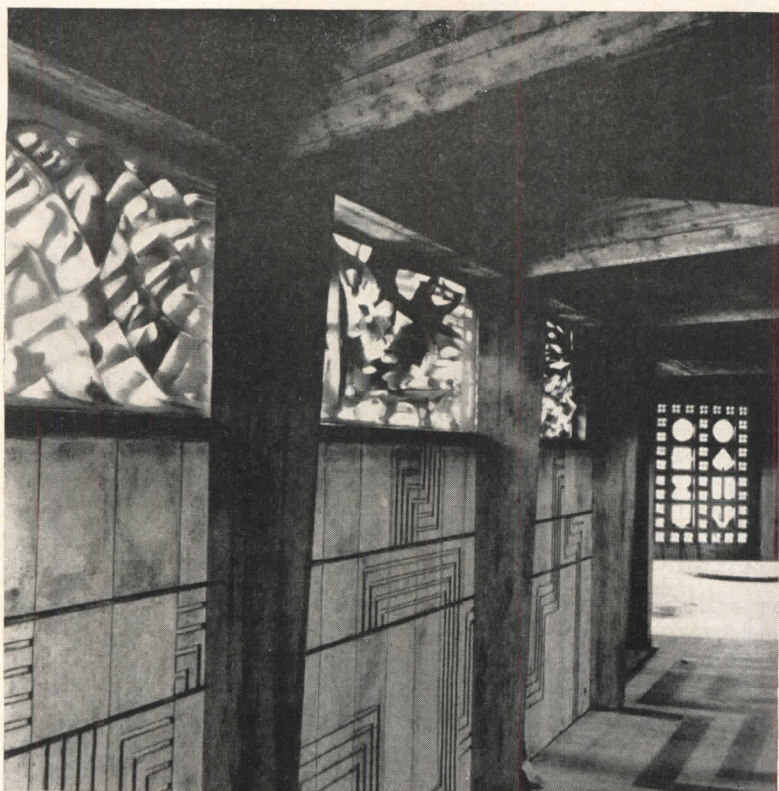
Interior of a church at Baccarat, France, combines form-board marking of columns with geometric pattern of precast slabs, the intertwined shapes of concrete and glass windows, and a pierced slab (background)
