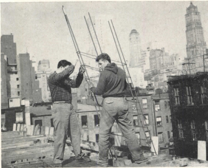
Reinforcing cage for column is lowered into form. Column and spandrel reinforcing was fabricated on the job. Below: Welded wire fabric in 19 combinations of wire spacing, gage, mat size, et cetera, is hoisted by crane, laid on previously-placed \frac{3}{4} -in. high "chairs"
