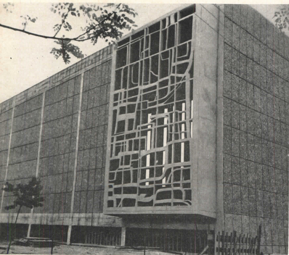
Glass-concrete window of St. Joan of Arc Church contrasts externally with exposed aggregate facings and internally with smooth, simple wall slabs
