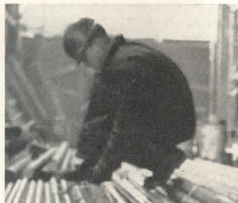
Prompt Delivery on the job site meets tight production schedules.
