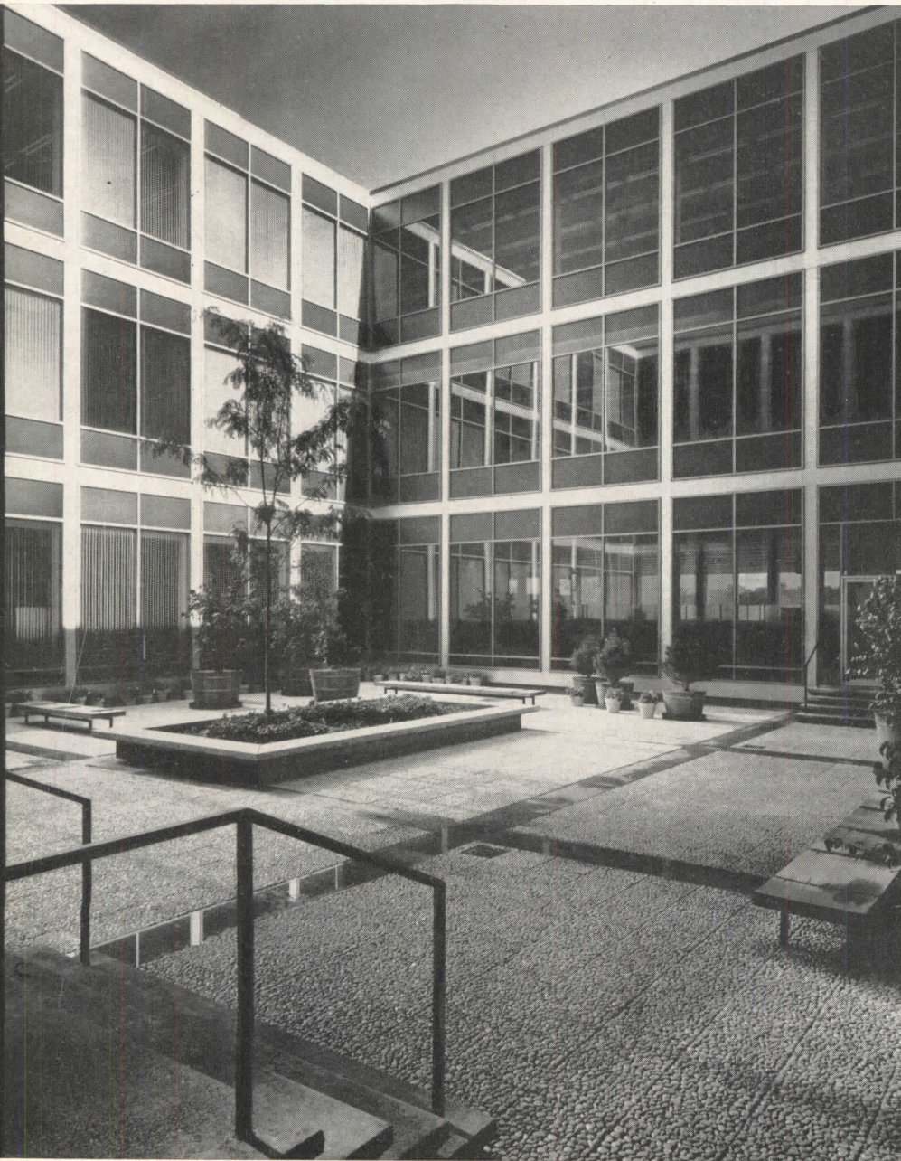
Main office area overlooks large court on first level roof. Court is completely enclosed on four sides by the aluminum and glass curtain wall, and provides additional daylight for offices
