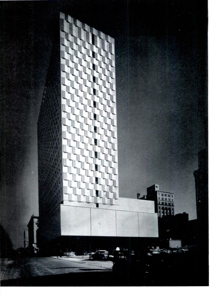
The view above shows the elevation of the building that faces the parking lot at the rear. The wall for this façade has been handled differently than the other three (page 189) since it faces the blazing afternoon sun. Windows have been reduced to a minimum in order to cut down the air conditioning load
