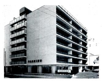
This mechanical garage, the Dundas Square garage, John B. Parkin Associates, Architects, is in Toronto, Ontario and uses a Pigeon Hole system
