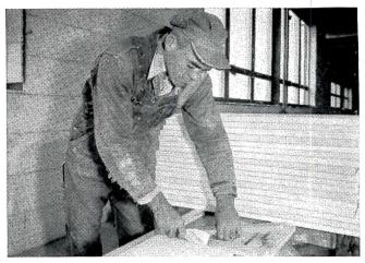
a mortar trowel. Not only does Styrofoam cut easily, but the cut surface is as smooth as if done by machine. This facilitates working around pipe, conduit, duct work, etc."
