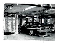
An example of the spare design possible with mechanized garages, the Tower Parking Garage in Columbus, Ohio, Tibbals-Crumley-Musson, Architects, uses a Pigeon Hole machine. Rising 88 ft above street level it is the tallest lift-slab structure in the U.S. Center: Top view showing elevator machinery. Lower: Ground floor view showing the pickup dolly of the parking machine in operation
