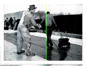
Lexsuco's semi-mechanical method is fast for medium or small jobs. Ribbons of adhesive are applied with spreader and rolled into a solid coat for securing Koroseal. Then insulation is embedded into the ribbons of adhesive spread over the Koroseal. It's like a production line! A manual method also is practical for small jobs using pouring can instead of spreader.
