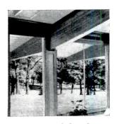
Cantilevered glulam beams extend the roof to form a canopy which protects the window areas from the sun. Classrooms receive natural light from three sides.
