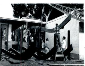
Nailed laminated beams form roof structure for seminar room being added to existing structure at CalPoly
