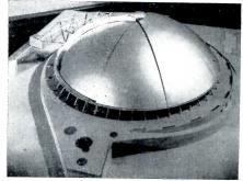
Stainless steel dome, 415 ft in diameter, has eight movable sections, two fixed
