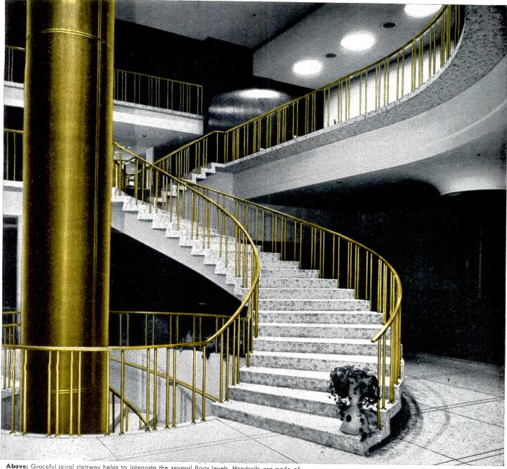
**Above:** Graceful spiral stairway helps to integrate the several floor levels. Handrails are made of formed Red Brass strip, reinforced with rectangular Red Brass rod, and the balusters are tubular Red Brass sleeves over a round steel rod. The column is enwrapped with woven bronze wires that have been partially colored to give a pleasing black and gold effect.
