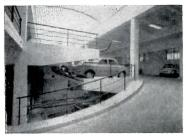
Fig 5 STAGGERED FLOOR, DIVIDED, TWO-WAY
