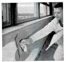
"PLASTERING DIRECTLY over Styrofoam eliminates complete operation of lath installation, permits substantial savings in cost. Styrofoam has the flexibility to give with expansion and contraction, provides a firm base for plaster."
