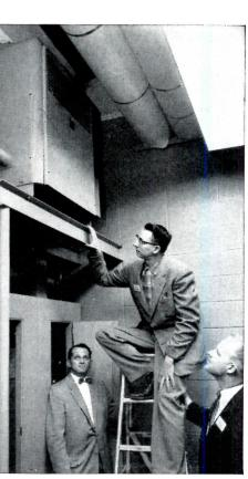
Robert Lichtenthal, James A. Reil, Ferguson Electric Construction Co., Electrical Contractors, and Charles Hansen discuss quietness and space-saving features which permit installation of Westinghouse 225-kva DT-3 dry-type transformer near office machines to which it supplies 120-v power.
