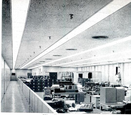
Ribbons of light-Sylvania recessed troffer lighting can be mounted in continuous rows and spaced for high lighting levels in modern business offices.
