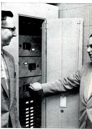
James Reil and Robert Lichtenthal check one of the two Westinghouse CDP panelboards which distribute 120 volts to the office machines from the Westinghouse 225-kva DT-3 dry-type transformer.
