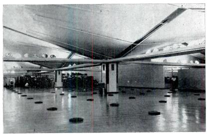
1500 access holes at 10- $\frac{1}{2}$  ft centers in the manufacturing floor slab make available any service at any point. Services include natural gas, some rare gases, water, electricity, communications and comfort conditioned air
