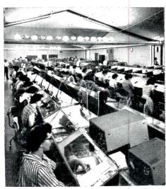
Extreme care in transistor assembly is exemplified by use of dry boxes in which humidity is limited to 12 per cent instead of 20 per cent as in room atmosphere itself
