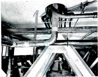
Above: As many as 16 different utilities are piped through one access hole. In a sense, space frame is a "basement" in the middle of the building. Openwork structure permits freedom of arrangement for equipment and accessibility for maintenance. At exterior, space frame has access doors to admit large equipment.
