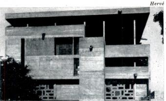
In 1956 LeCorbusier used boldly projected concrete pipespouts to drain the flat roof and raised verandahs of a house at Hyderabad, India
