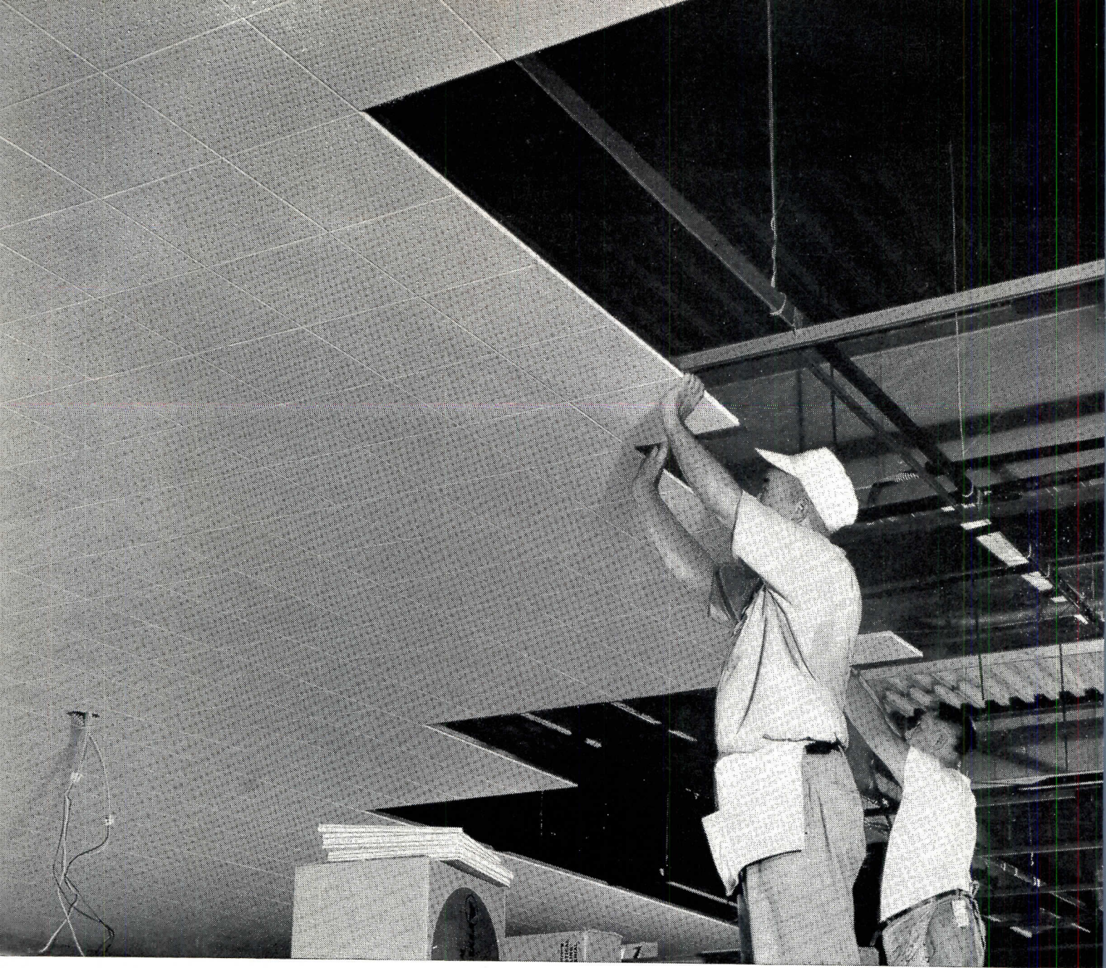
These mechanics are installing an Armstrong Minatone Ceiling under ideal job conditions. Electrical work has been located, and the building is thoroughly dry.
