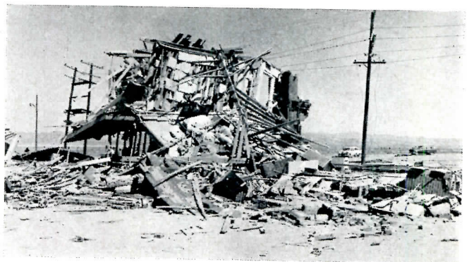
BRICK — Unreinforced two-story house; 5 psi overpressure
