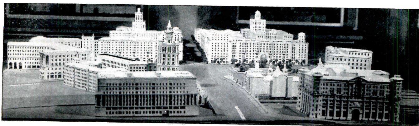
Model of the future Byelorussian Railway Station Square; name of architect not available
