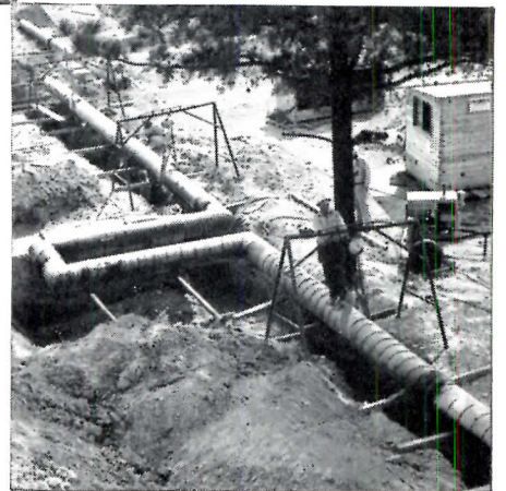
Tested and ready for lowering long lengths.
