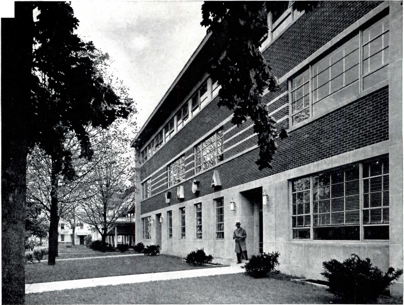
The new Y.M.C.A. in Stroudsburg, Pa., was designed by Rinker and Kiefer, architects. General contractor: Paul L. Edinger. Both are Stroudsburg firms.
