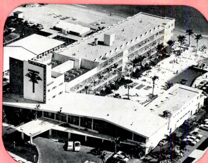
Thunderbird Motel, Miami Beach, Fla.; Archt.—Norman Giller & Assocs., Miami Beach; Contr.—Taylor Construction Co., Miami; Engr.—Jules Channing, Miami; Pozzolith Ready-Mixed concrete—Maule Industries, Inc. & Acme Concrete Corp.
