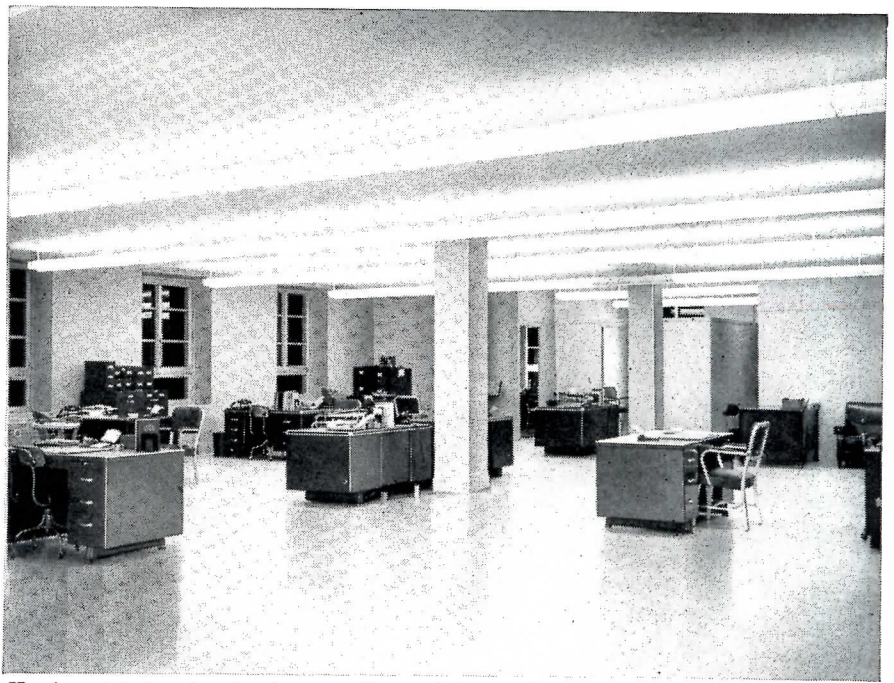
Here's an interior view showing a small part of the installation of Gold Seal Inlaid Linoleum. Actually, about 3½ acres of floor space are covered with this ⅛" burlap-backed "Veltone."
