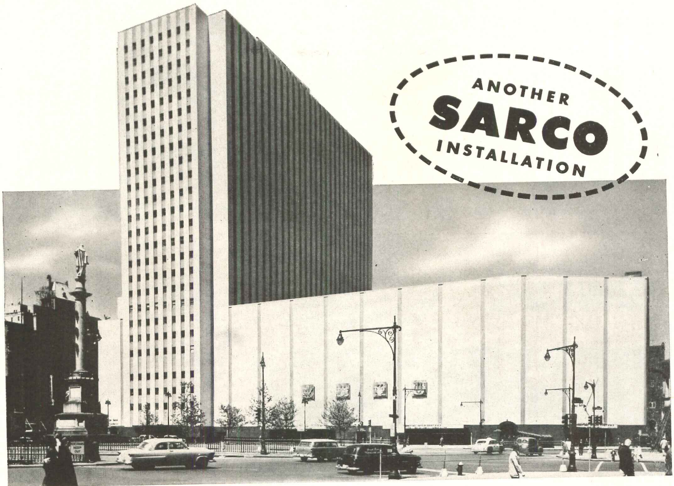
The New York Coliseum, New York City. Owners: Triborough Bridge & Tunnel Authority. Architects: Leon & Lionel Levy. Mechanical Engineers: Guy B. Panero Engineers. Heating Contractors: Almirall & Co., Inc.
