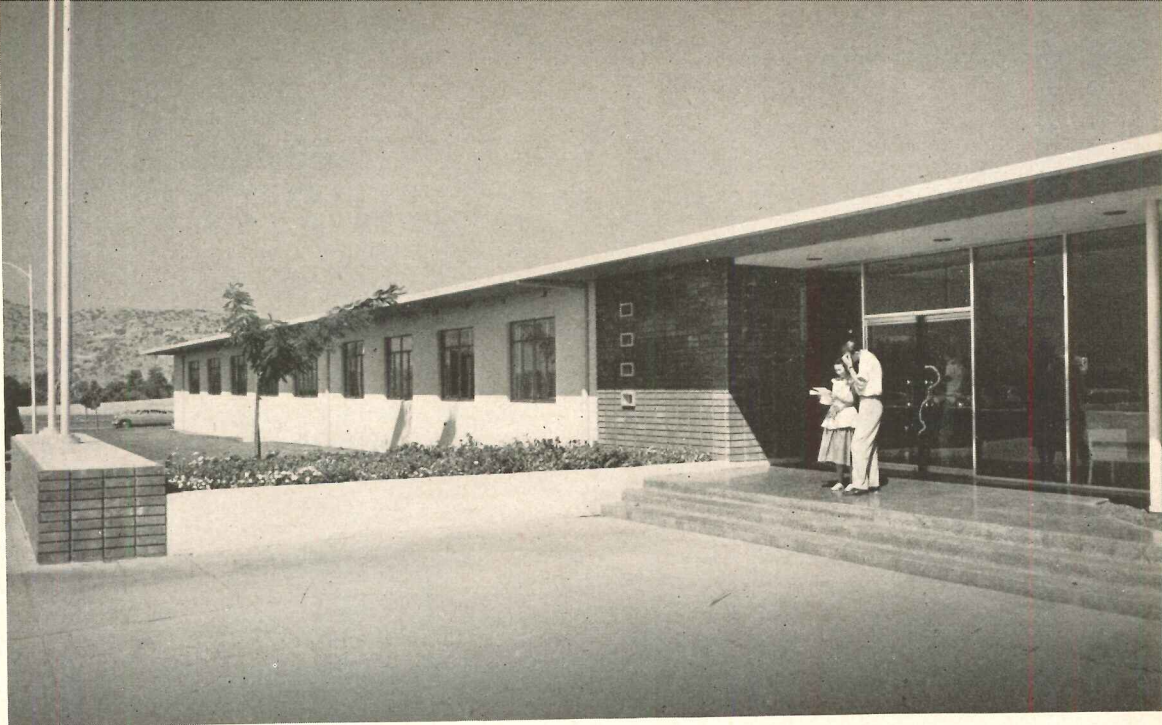
The Administration Building sets a note of spaciousness with a wide entrance plaza and planting beds
