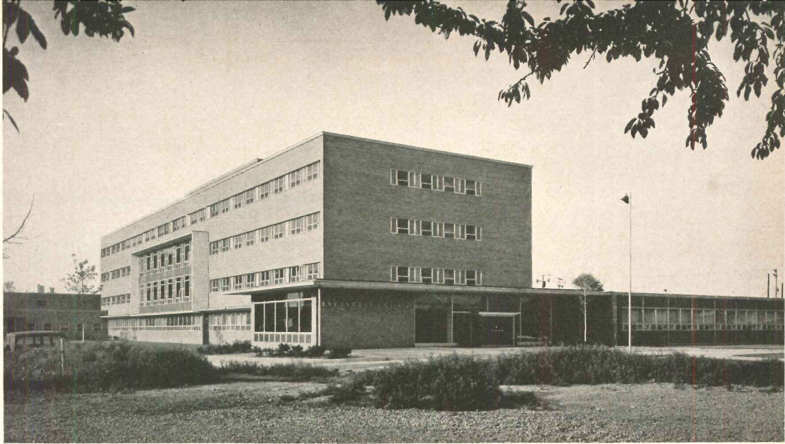
General exterior view, from right-hand end of plan (opposite page). Entrance serves outpatients
