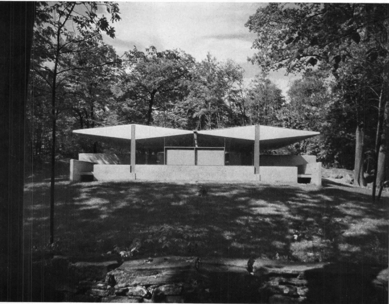
ULRICH FRANZEN, ARCHITECT AND OWNER. RAYBECK INC., CONTRACTOR
