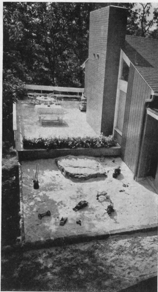
Space outside the McGranahan house is organized into areas of varying use: living deck, dining terrace, service area with children's playground, quiet areas off the bedrooms. Lights below deck shine on trees around house at night
