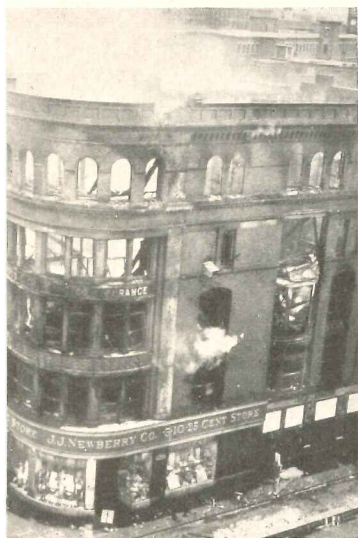
Central Block Building, Lowell, Mass. Burned March 17, 1955. Loss: $561,000. Contributing causes: no automatic detection, unsprinklered areas, unenclosed stairwells and elevator shafts.
