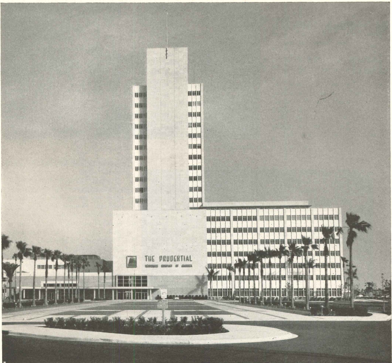
Thousands of Bethlehem High-Strength Bolts were used to join structural members in framework for new Prudential office building in Jacksonville, Fla. Architects: Kemp, Bunch and Jackson. Contractor: Daniel Construction Company of Alabama. Fabricator and Erector: Ingalls Iron Works Company.
