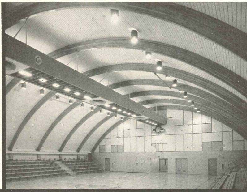
HIGH SCHOOL GYMNASIUM . . . MAYNARD, MINNESOTA Architects: Haarstick Lundgren & Associates, Inc. • St. Paul, Minn.
