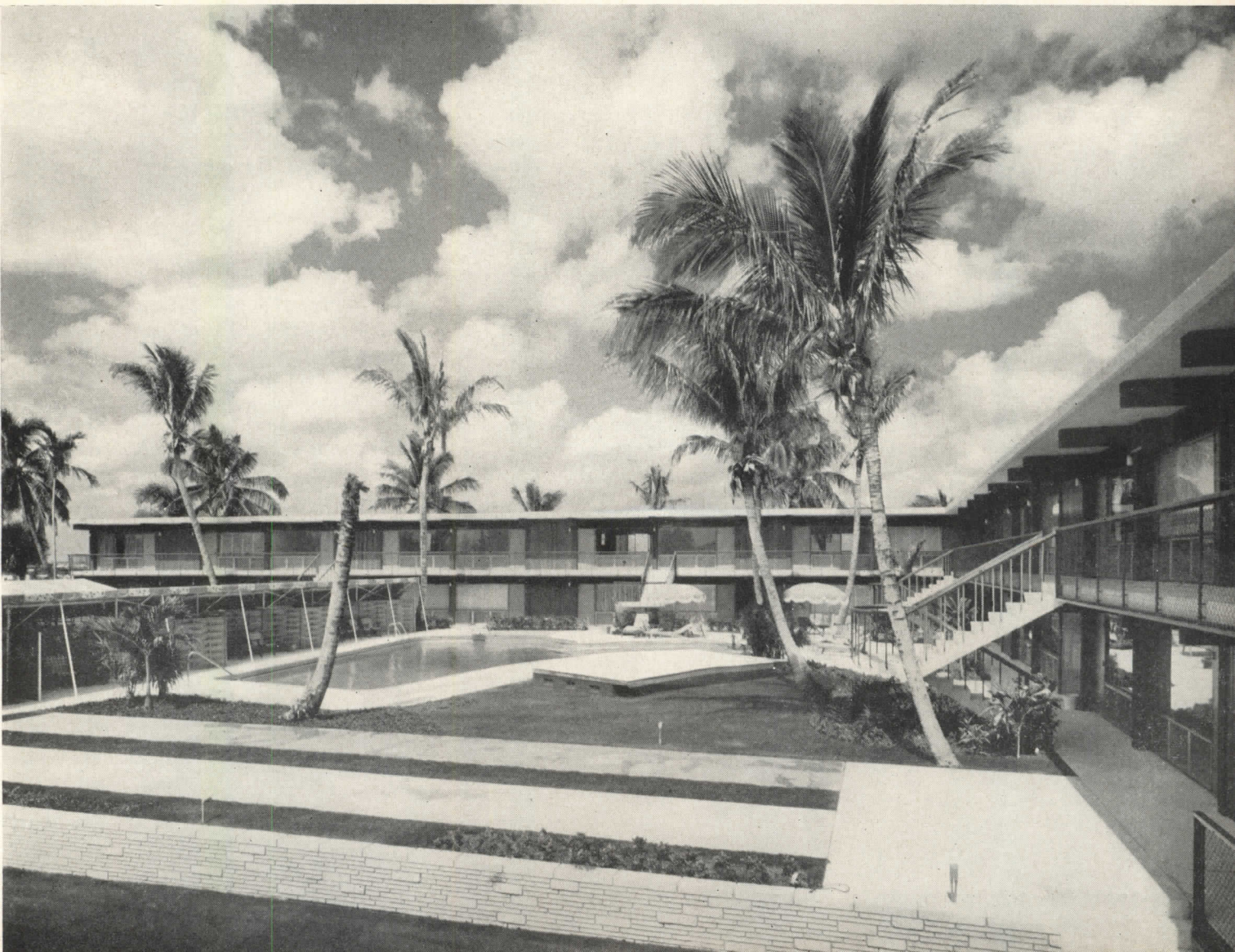
To combat high cost of accommodations at resorts this cooperative motel-apartment-hotel was built recently at Fort Lauderdale, Fla., Robert Hanson, Archt. (Alexandre Georges)
