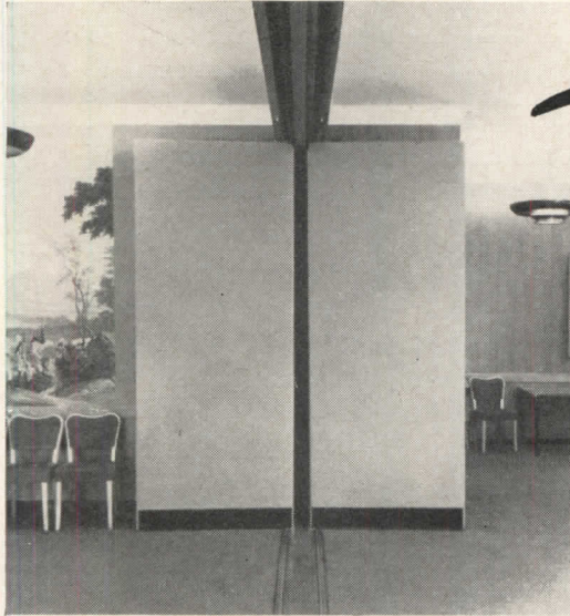
Fairhurst double wall units stacked at side of room.
