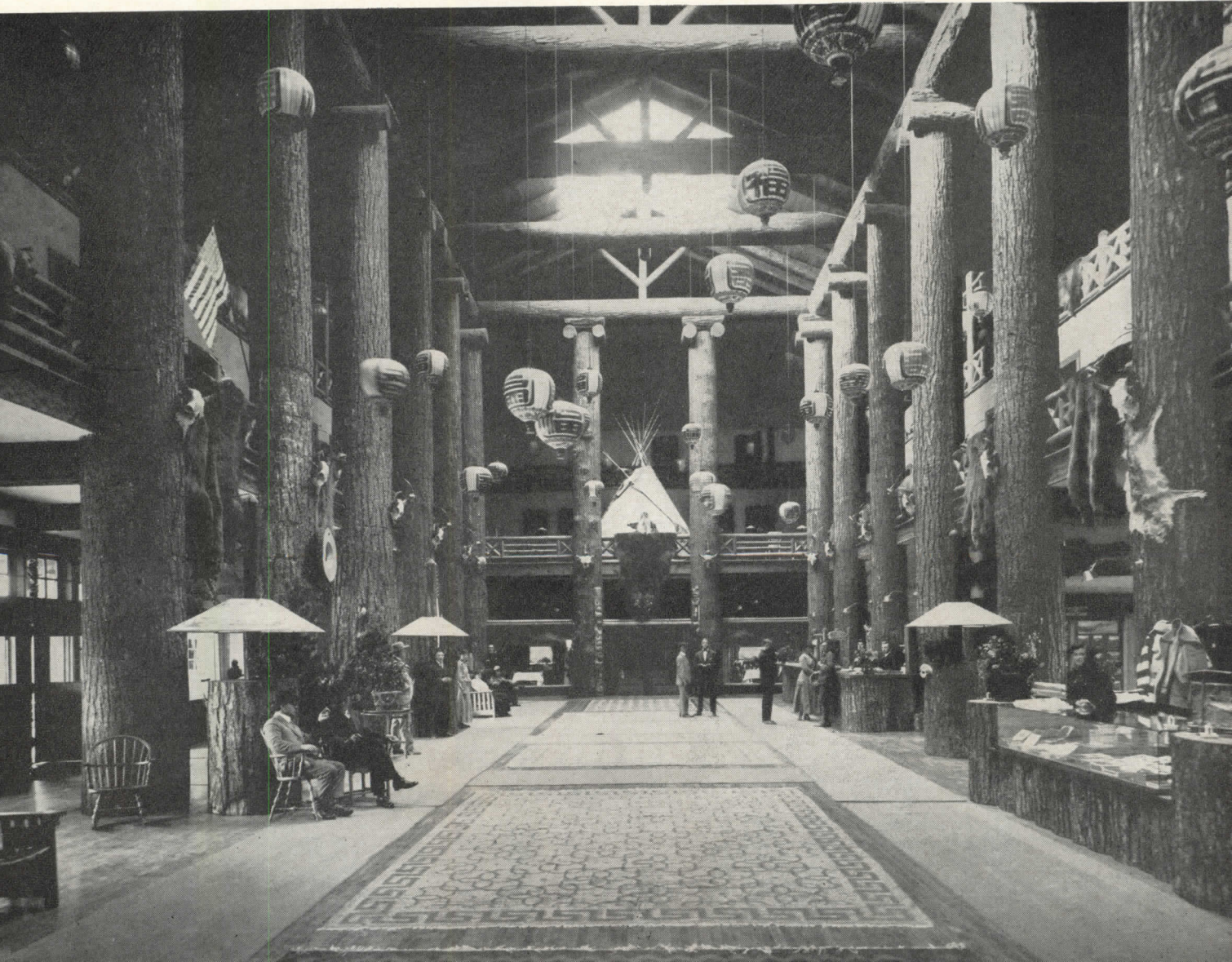
Lobby, Glacier Park Hotel, Montana; note Ionic columns formed of log sections (Culver Service)
