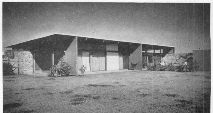
Structure. Post and beam, with structural elements exposed throughout; 4 by 10 in. beams on 7 ft centers form module for glass sliding panels on south and fixed glass and glass lower panels on north; roof deck exposed and stained a rich brown to form the finished ceiling
