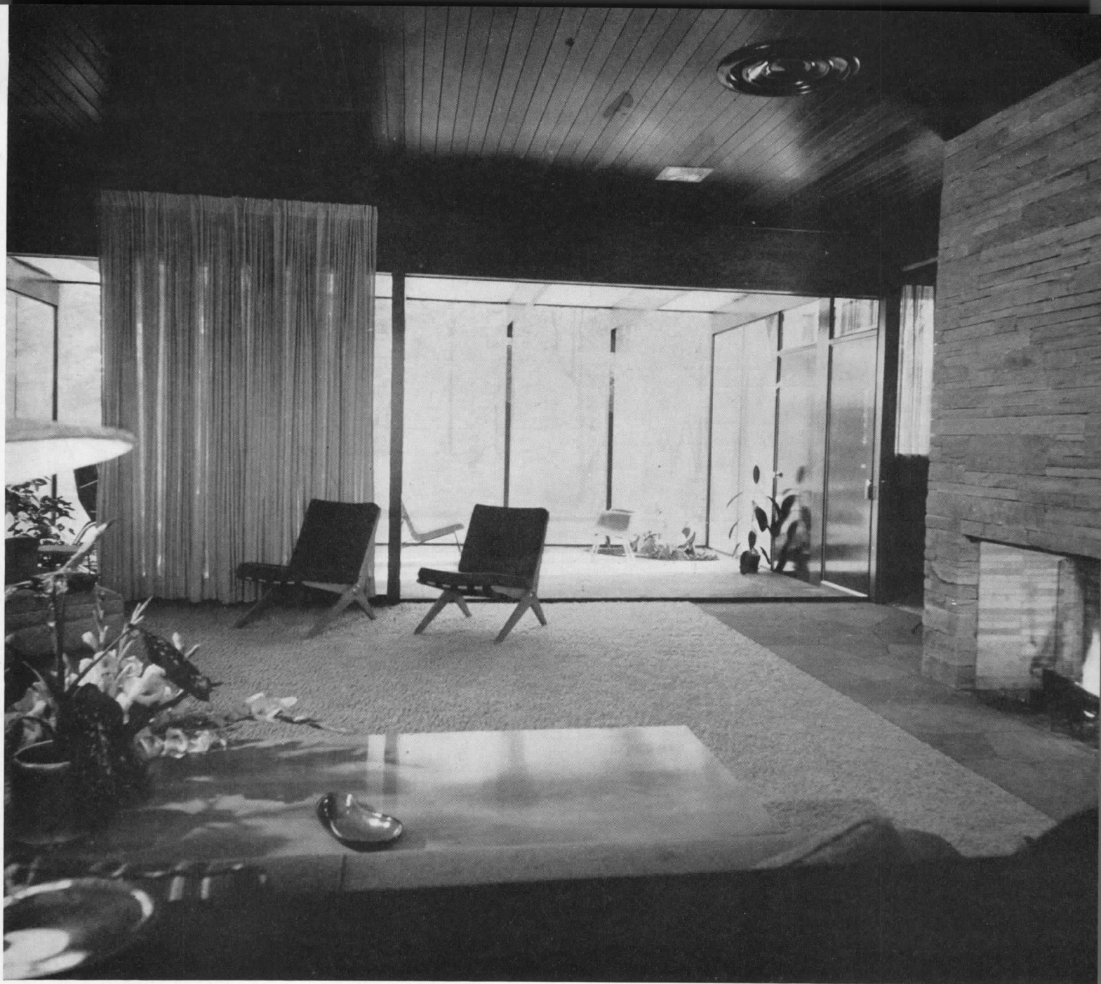
Warm Materials. Construction is wood frame on concrete slab with exterior siding of T&G redwood in contrasting vertical and horizontal treatments; in living area ceilings are redwood, walls are white plastered; chimney is flagstone, as are floors in entry and screened porch
