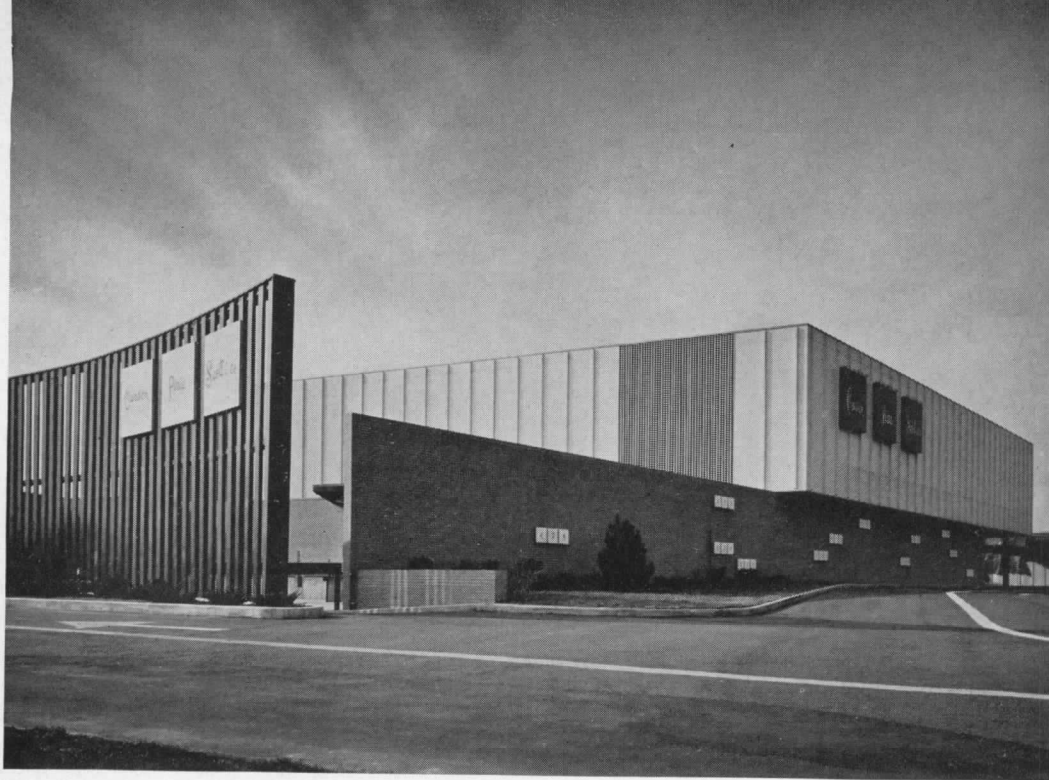
Department store loading area is concealed by a curving screen of wooden louvers, above. The second floor volume is covered with white glazed brick; the first floor with red face brick
