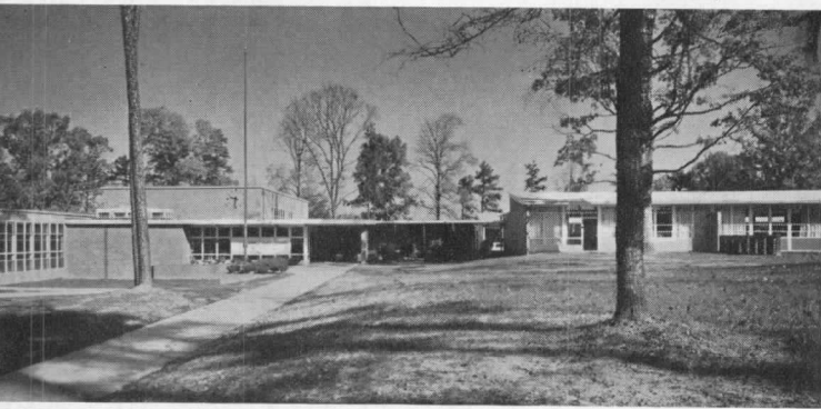
Double Oaks Elementary School, Charlotte Public School System; A. G. Odell, Jr., Architect
