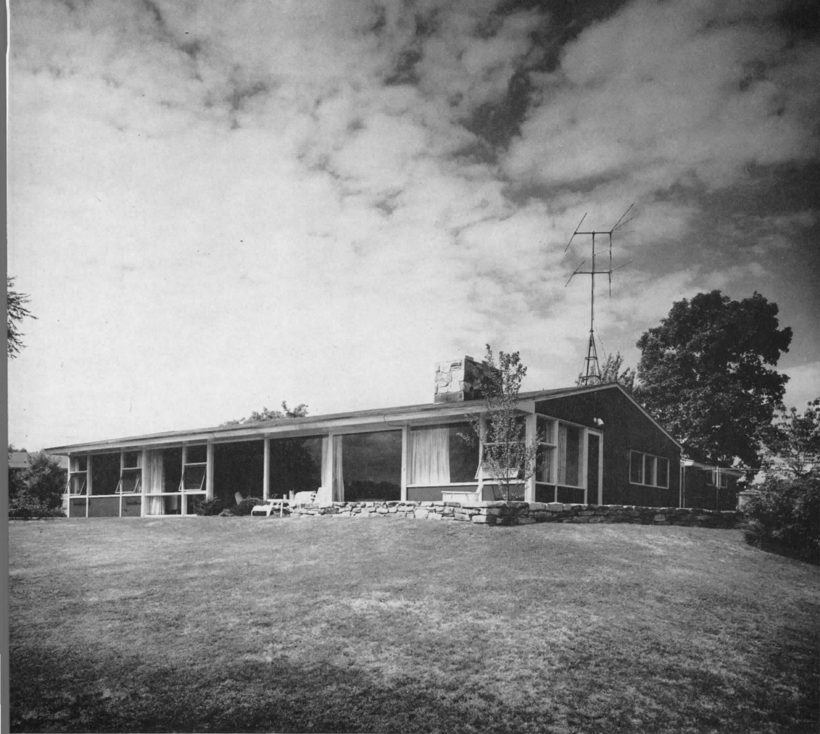
Site Relationship. Site is large, with a long gradual slope at rear which low pitch of roof echoes; living room has floor-to-ceiling glass wall which extends room to far corner of site. Materials. Vertical T&G siding and painted (red) plywood panels on exterior; concrete floors
