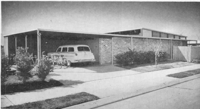
Structure. Post and beam, with structural elements exposed throughout; 4 by 10 in. beams on 7 ft centers form module for glass sliding panels on south and fixed glass and glass lower panels on north; roof deck exposed and stained a rich brown to form the finished ceiling
