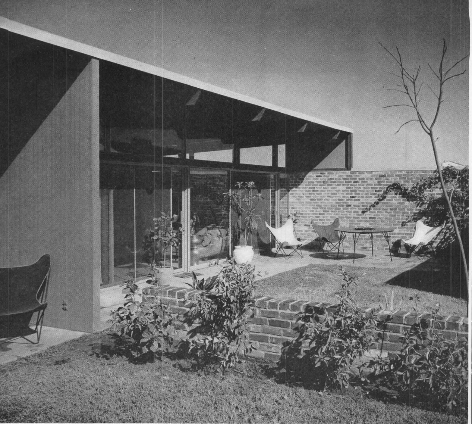
Structure. Post and beam, with structural elements exposed throughout; 4 by 10 in. beams on 7 ft centers form module for glass sliding panels on south and fixed glass and glass lower panels on north; roof deck exposed and stained a rich brown to form the finished ceiling
