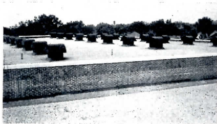
Skylights in Schools — Corrugated translucent structural panels of fiberglass-reinforced plastic illuminate this corridor so that it can be used for exhibitions or for extra schoolroom space. Resolite Corp., Zelienople, Pa.
