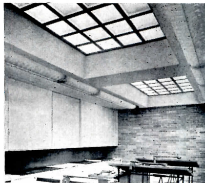
Skylights in Commercial Buildings — Glass blocks in the roof of this architect's office provide plenty of daylight for drafting. Cast into a steel-reinforced concrete grid, the Skytrol blocks are good insulators. Pittsburgh Corning Corp., 1 Gateway Center, Pittsburgh 22, Pa.
