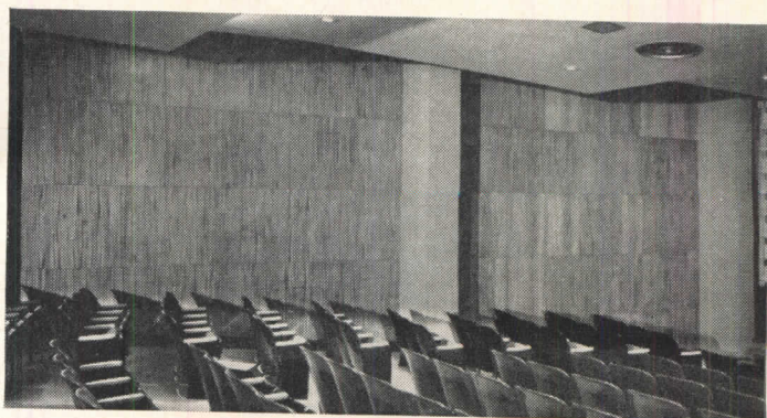
AFRICAN MAHOGANY WELDWOOD was used to panel auditorium walls. Notice the dramatic staggered grain effect made possible by this tier arrangement. Each tier is approximately 3' high.
