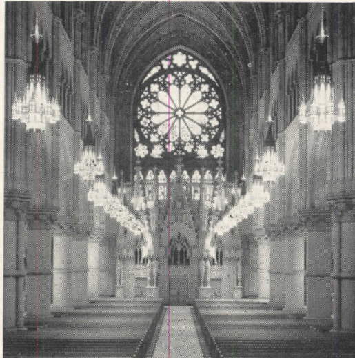
View from altar looking toward rose window over main entrance.
