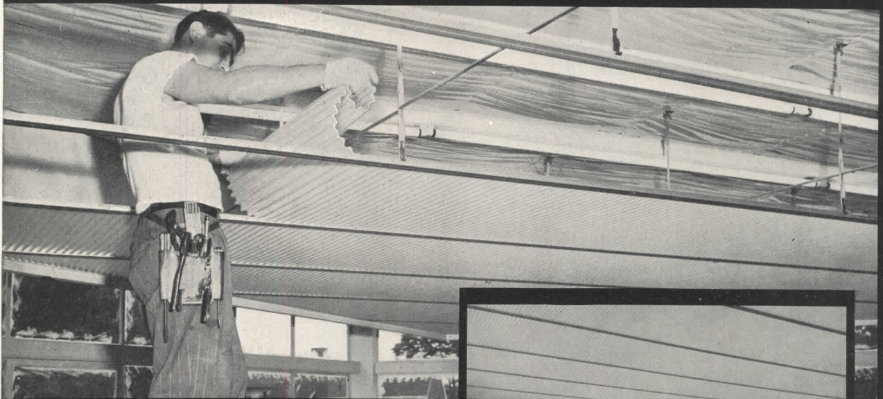
Workman slides continuous corrugated ULTRON rigid vinyl sheeting into supporting channels in new classroom for Franklin Elementary School, West Newton, Mass.
