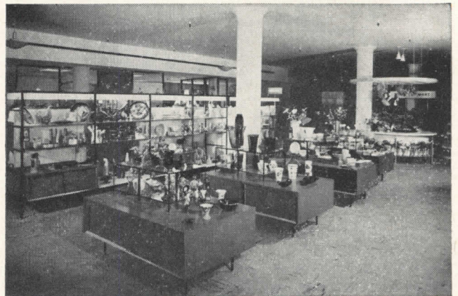
Overhead ductwork and outlets blend with the décor of Macy's—New York—gift department in their Herald Square store. Interior architecture: Copeland, Novak & Associates.
