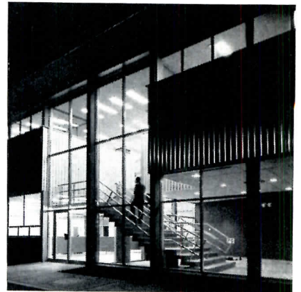
Three views of a new bus depot recently built in Westminster, B. C., by the British Columbia Electric Railway Company Ltd. Fluted facings and spandrels are of aluminum sheets which have been polished and anodized. Architect for the building was Percy C. Underwood of Vancouver, B. C.
