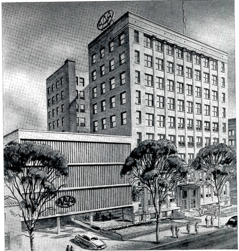
NEWLY REMODELED American Automobile Association Building in Washington, D. C., is air conditioned by 3 G-E Packaged units on each floor. Architect for remodeling was A. R. Clas; George H. Riggs, Jr., associate. Consulting engineers: Lanier & Levy. General contractor: Wm. P. Lipscomb Co. Mechanical contractor: Morris and Eagan Co.
