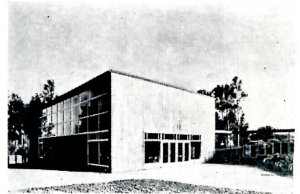
Award of Merit—Highlands (Elementary) School, Millbrae, Cal.; John Lyon Reid, Architect
