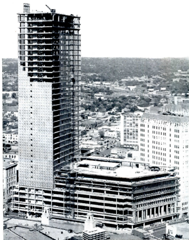
Progress shot, November 1, 1953
