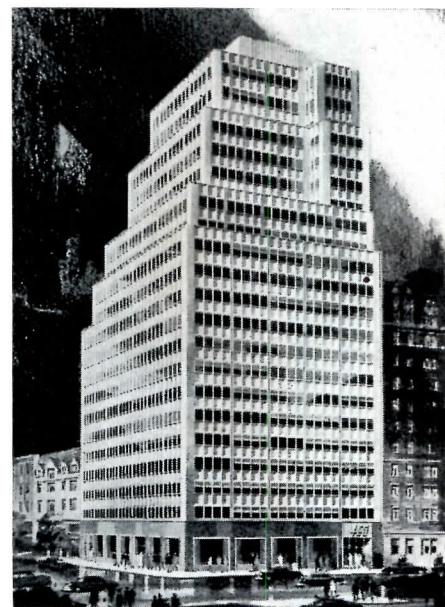
Twenty-two story air conditioned office building being erected at Park Avenue and 57th Street, N.Y.C. will have an aluminum skin. Architects: Emery Roth and Sons
