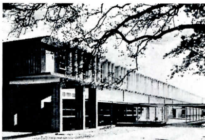
Award of Merit—El Rancho High School, Whittier, Cal.; William H. Harrison, Architect
