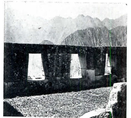
Above: at Machu Picchu, three windows of typical trapezoidal shape. Below: detail of stonework at Ollantaytambo; so closely fitted that it is impossible to insert a knife between the blocks
