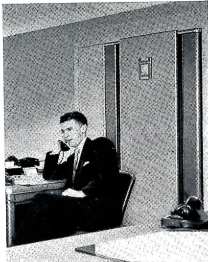
IN-SPACE APPLICATION of 5-ton G-E unit. It air conditions large membership room in which it is located plus other offices. Note streamlined vertical air inlets.
