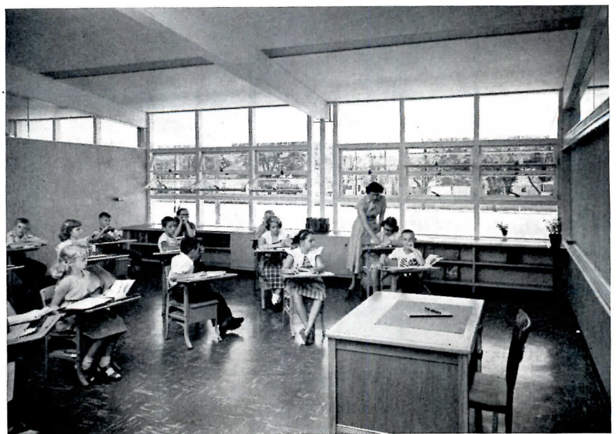
Both schools are framed with heavy laminated wood beams on pipe columns, have 12-in. cavity brick exterior walls; projected steel sash; built-up, heat-reflective roofs; stained fir plywood partitions. Heating systems are low-pressure hot water circulated through wall convectors and panels in the concrete floor slab; controls are electronic
