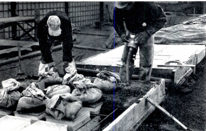
CONCRETE is kept on the dry side (3" maximum slump) and is vibrated to eliminate voids in the reinforced concrete web. Sandbags eliminate possibility of block disalignment during vibrating.
