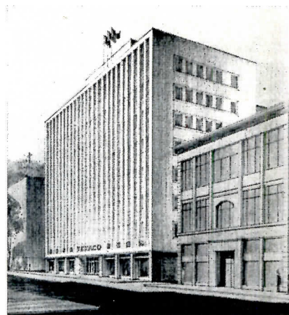
McColl-Frontenac Oil Company Ltd. also plans a new office for Montreal. Construction of the T-shaped building will be of reinforced concrete, with buff brick facing and granite trim. Architects are Barott, Marshall, Montgomery and Merrett
