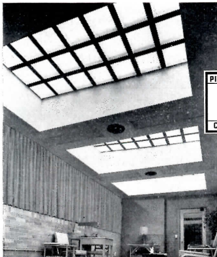
HERE'S the finished panel. After seven days of wet curing, the SKYTROL panel is ready for long-life, maintenance-free service.
