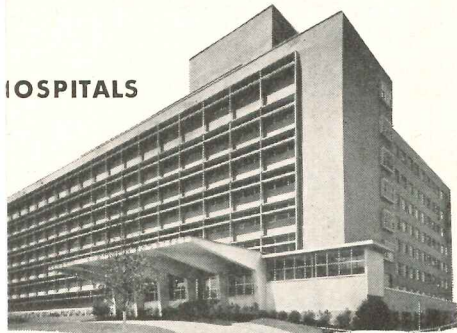
Georgia Baptist Hospital, Atlanta, Ga. Architects: Stevens & Wilkinson, Inc.
