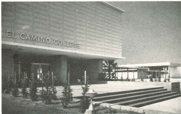
El Camino College, California. Exterior concrete painted with Wesco Durasite Marsh, Smith & Powell, Architects, Los Angeles
