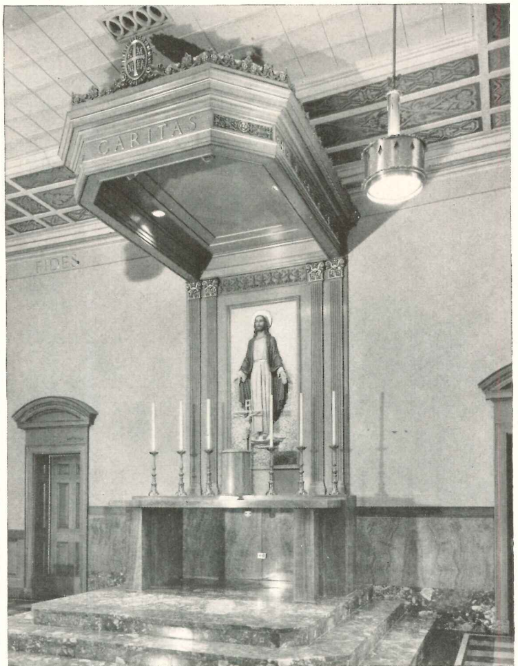
Reredos and Tester, Main Chapel Altar, Cardinal Stritch Retreat House, Mundelein, Illinois—Architects, McCarthy & Smith, Chicago
