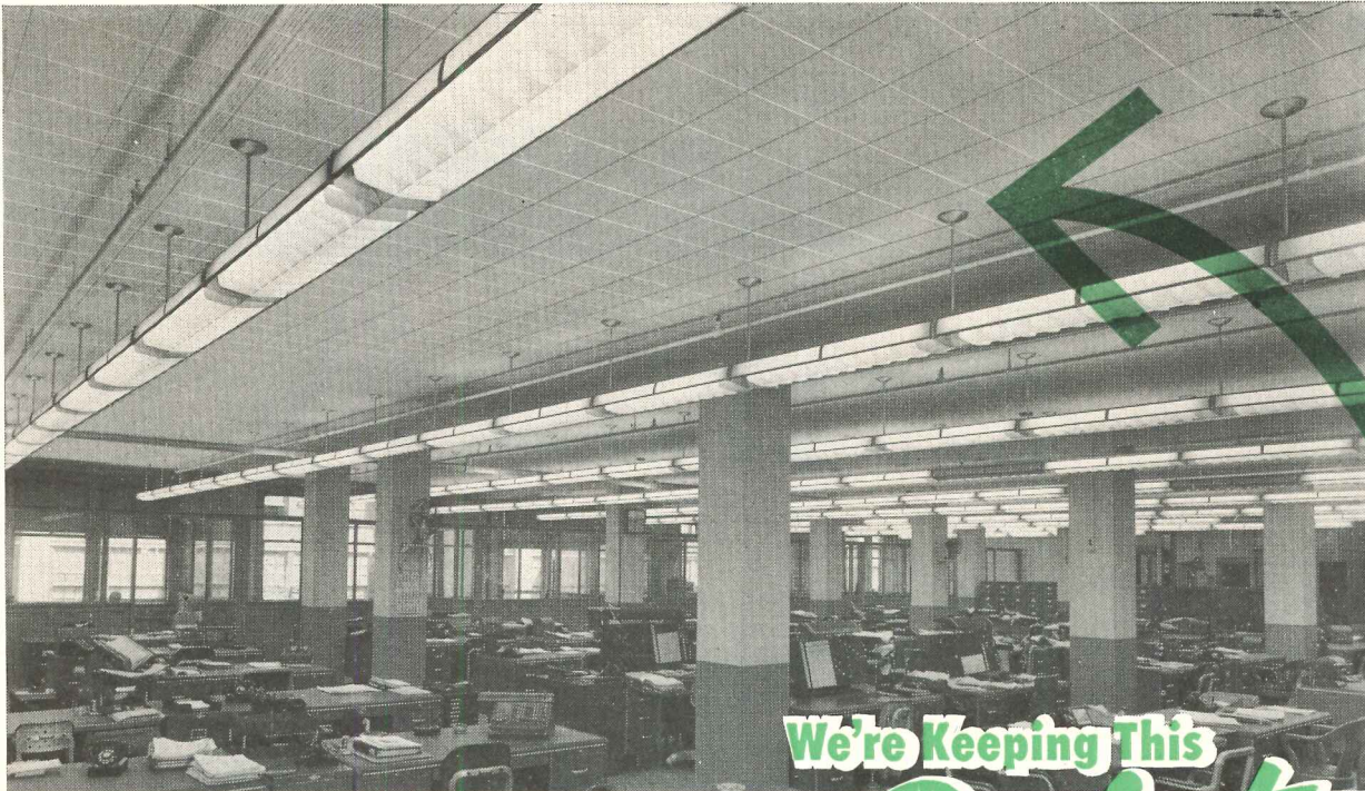
Offices of B. F. Goodrich Company, Cleveland. Simpson Acoustical Tile installed by The Mid-West Acoustical & Supply Company, Cleveland
