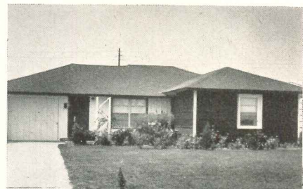
HOUSTON, TEXAS. All 84 units in McGregor Terrace Addition are built with Rusco.
