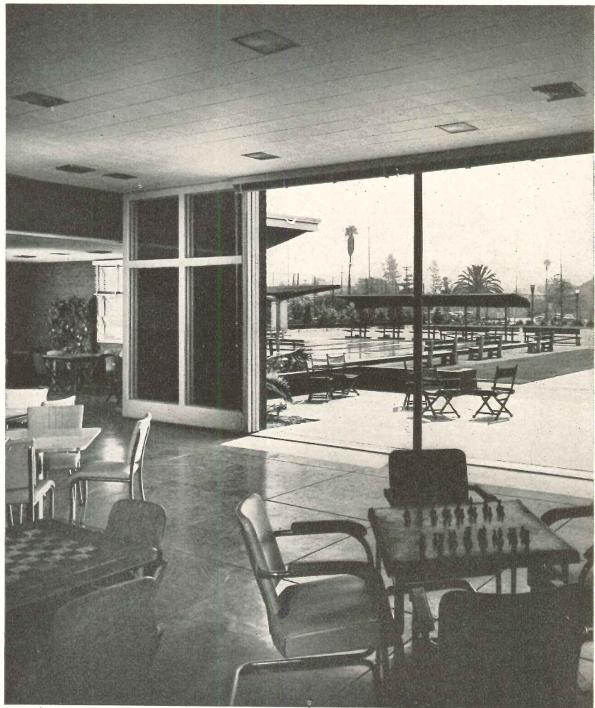
Far right: concrete-based columns, slatted at top to receive cantilevered beams, with redwood louvers spaced and sloped at carefully controlled angles in opposite directions at north and south shelters, cut down summer sun on shuffleboard courts and secure maximum winter sun
