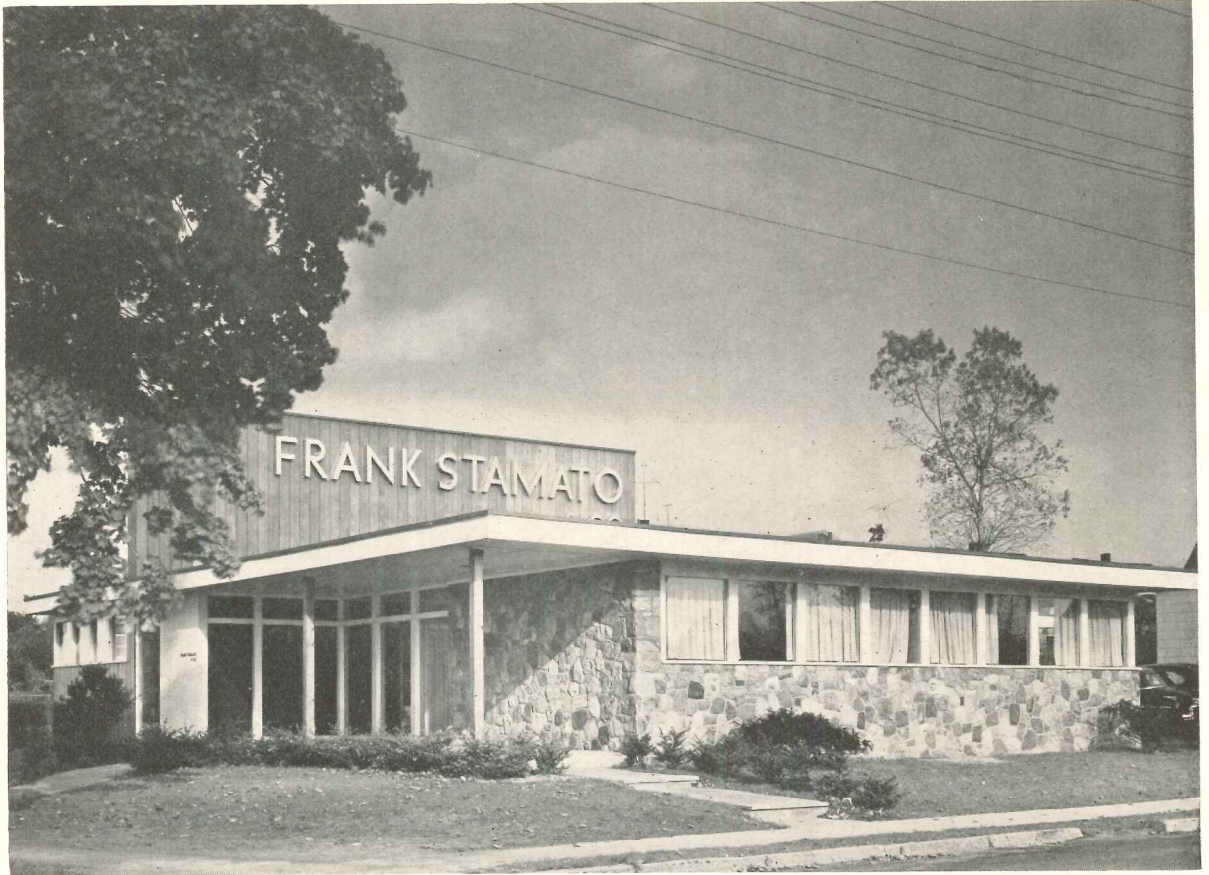
FRANK STAMATO & CO. OFFICES
