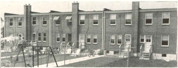
BALTIMORE, MARYLAND. Rusco Prime Windows specified on all 87 units of Gebhart Housing Project.
