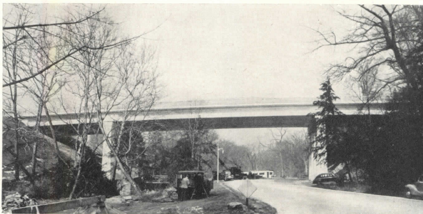
Above: first prestressed bridge to be started in this country was the Walnut Lane Bridge in Philadelphia. Below: the West's first, the Arroyo Seco Pedestrian Crossing, Los Angeles, Calif.
