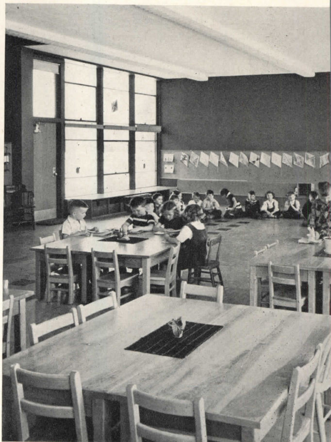
Kindergarten has bilateral window walls as well as clerestory at interior corner. Architects do not want to make clerestoried classrooms so high again; lowered 16 in., they would have scale better related to children, cost less
