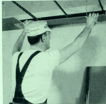
2. Now a piece of Gypsum lath is engaged by the starter clips. Plain or perforated 3/8" Gold Bond gypsum lath may be used. Handy clip cartridges are attached to lather's belt. Clips are made of strong wire.
