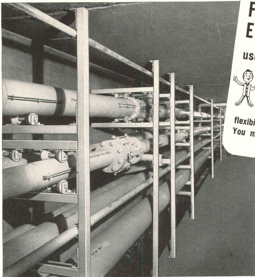
Unistrut steel channel and fittings, roller pipe supports and concrete inserts at work in a tunnel installation at G. D. Searle & Co., Skokie, Illinois, manufacturers of ethical pharmaceuticals.
