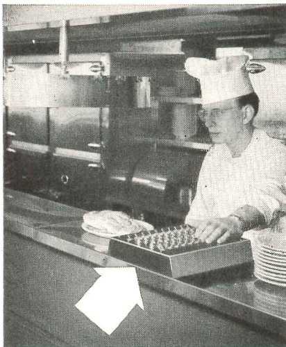
Arrow points to Type RC-20J Single Pole Toggle Switch Control Unit, with Jewel Bull's-Eye Lights and Chime Ringing Buttons operated by chef as order is ready. Waitress turns off switch as she picks up order, clearing lighted numbers from annunciator.
