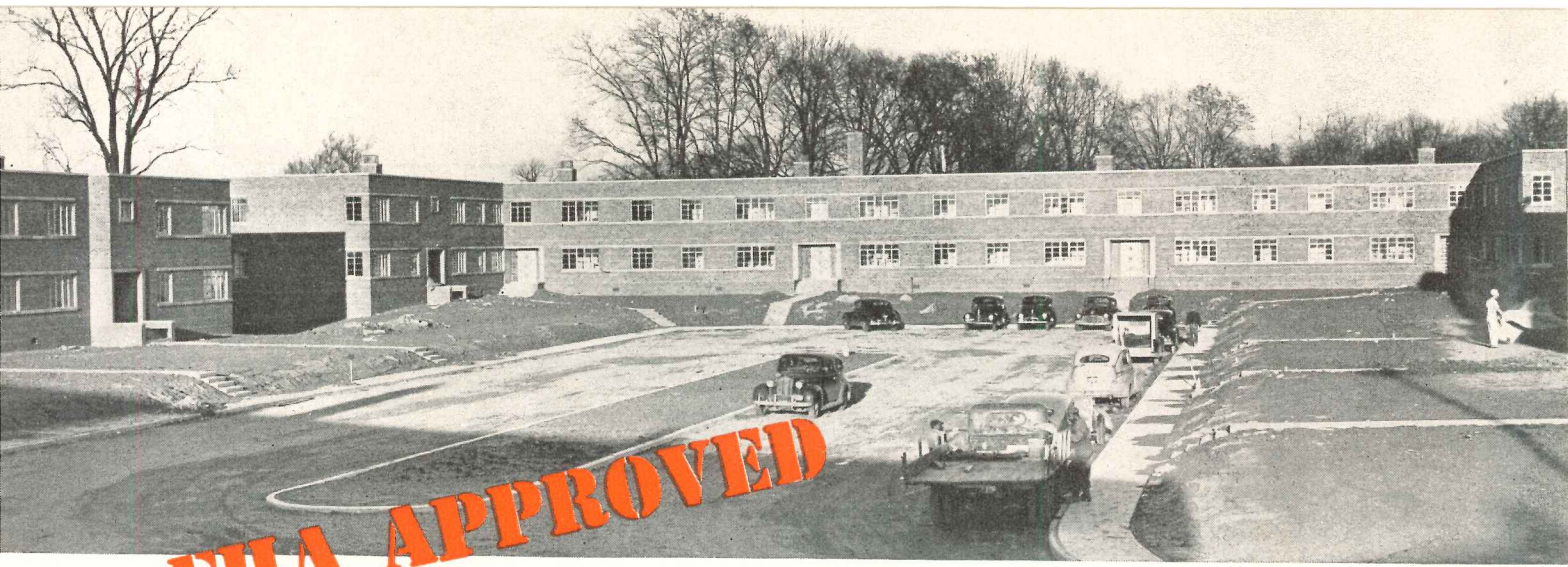
Partial view of Meadowbrook Apartments, Indianapolis, Indiana. Owners: Meadowbrook Sponsors. Architects and Engineers: Allen and Kelley. General Contractor: Mars Engineering, Inc. Heating and Plumbing: Freyn Brothers, Inc. Electrical Contractor: Hatfield Electric Co. All of Indianapolis, Indiana.
