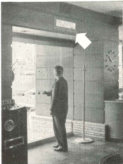
Entrance to Bob's Drive-in Restaurant in Eagle Rock, California, Type M-20 (20 number) with Chime. Cannon Annunciator over door is plainly visible to waitresses to indicate waiting orders.
