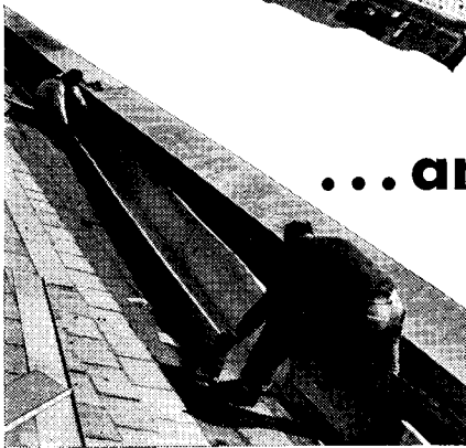
INSTALLING A RIVETED AND SOLDERED section of Monel Roofing Sheet in the built-in gutter of the Pentagon's outer perimeter. Fabricator, Rupertus Sheet Metal Works, Washington, D. C., reports: "Some of the gutters were 55 inches in girth, but Monel was easy to fabricate and install."
