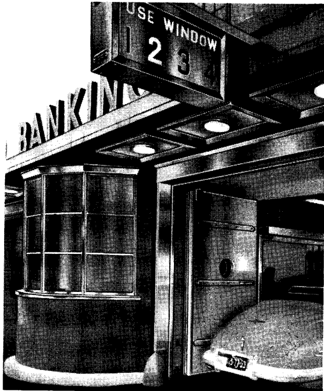
Drive-in banking installation
