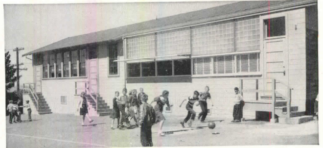
CALIFORNIA! For the extremely bright sun problem presented by Cragmont Test School in Berkeley, Insulux Glass Block (No. 352), with improved prism faces and special glass fiber screen inside, is used to improve classroom daylighting over old-style windows (extreme left). Architect: John Carl Warnecke, Oakland, Calif.
