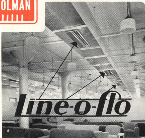
Illustrating use of individual "LS" LINE-O-FLO units set into exposed ducts in a large retail store and show room.
