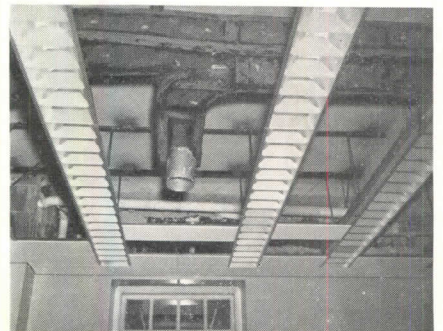
Above: lighting troffers support acoustic ceiling. Below: completed installation
