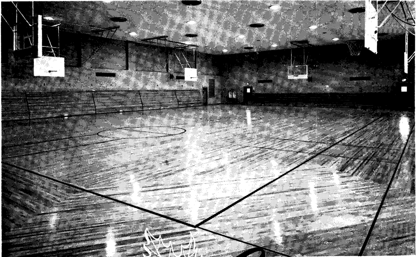
Floor of Northern Hard Maple, 80 x 100 feet, a dual-purpose innovation which combines gymnasium and roller-skating rink, at Archbishop Stepinac High School, White Plains, N. Y.—an interesting development in supervised recreation. Eggers & Higgins, Architects, New York, N. Y.
