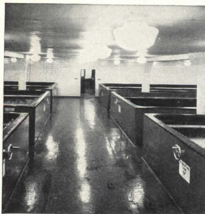
GRIESEDIACK BROS. Brewery, St. Louis—multiple-story closed fermenting tanks. Tanks, walkways, walls, stairways form completely monolithic structure.
