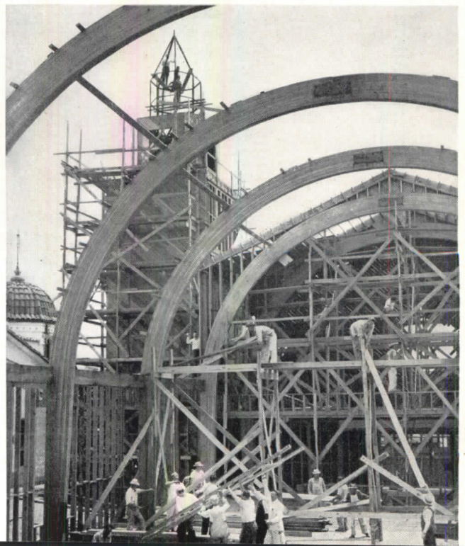
Left: three-hinged arches for high school, Barrington, Ill.; Perkins and Will, Architects. Right: Trinity Baptist Church, Santa Monica, Calif., uses five curved arches, 46 ft, 8 in. wide and 17 ft on center; Louis S. Gamble and Associates, Designer
