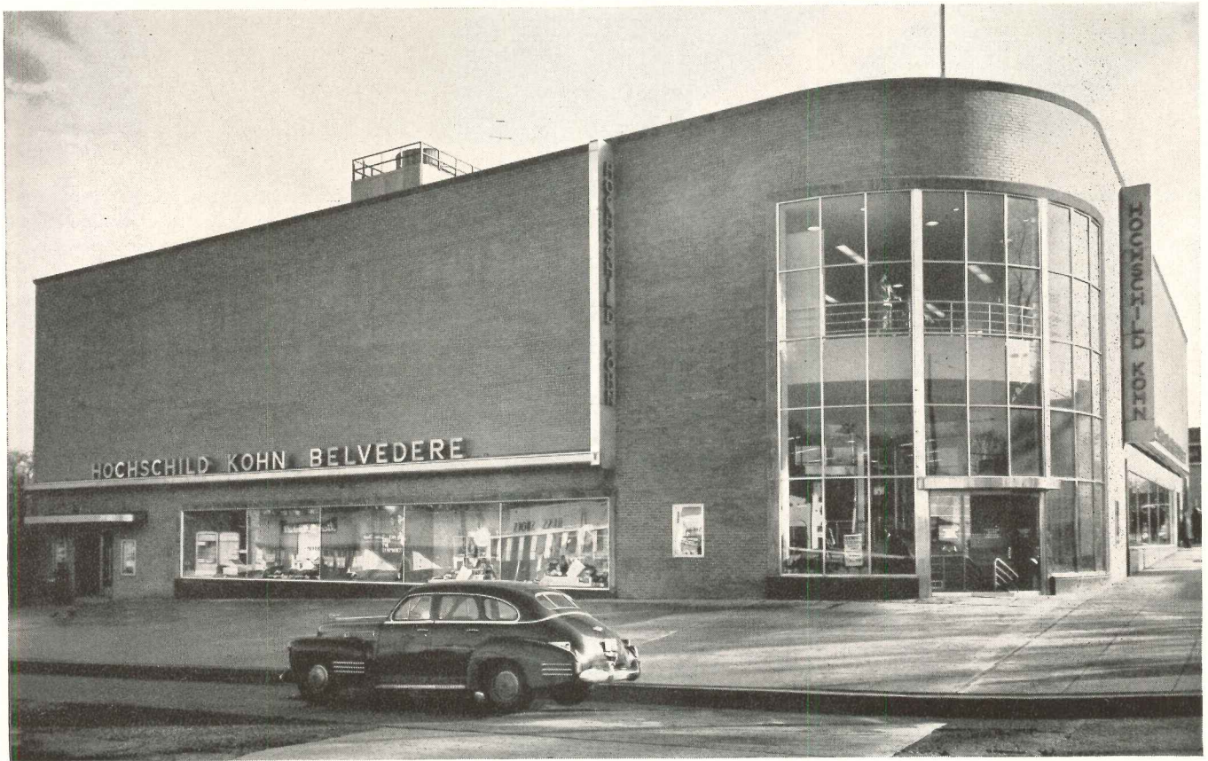
The new Hochschild Kohn store in Baltimore, Maryland. It was designed by the office of James R. Edmunds, Jr., Architects, Baltimore. Contractor: Morrow Brothers. Signs and storefront by: George R. Habgood Company, Philadelphia; Triangle Sign Company, Baltimore.
