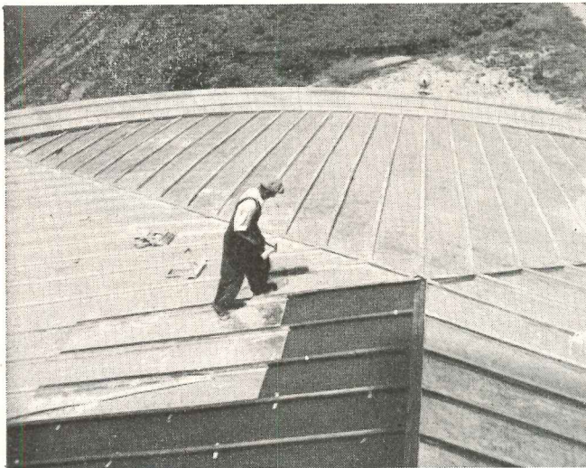
Back roof, where double pitched roof and dome roof meet.
