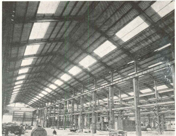
Corrugated Fiberglas -plastic sheets that can be sawed and nailed provide daylighting for Tulsa, Okla. industrial plant. Left: shows how sheets are fastened to steel rafters of entrance to mill building. Right: the translucent sheets used as skylights
