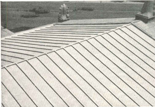
Finished double pitched roof on front.
