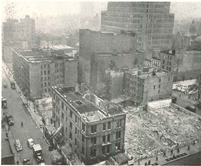
The Terminal site in October, 1948, during demolition proceedings
