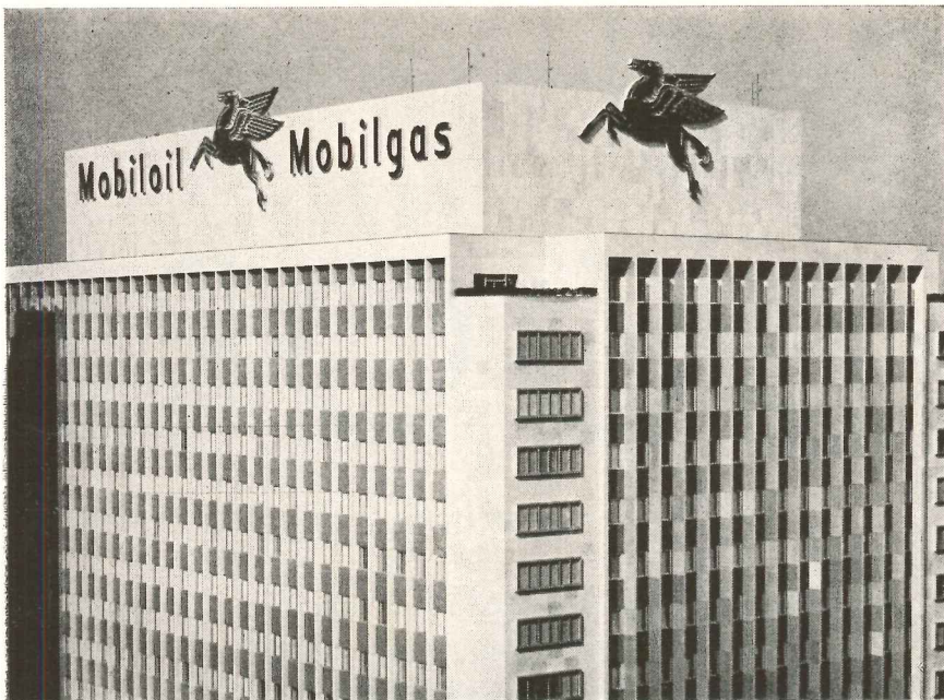
GENERAL PETROLEUM BUILDING, LOS ANGELES, CALIFORNIA
