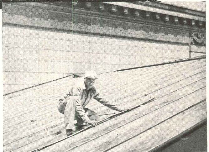
Installing caps on batten as roof nears completion.
