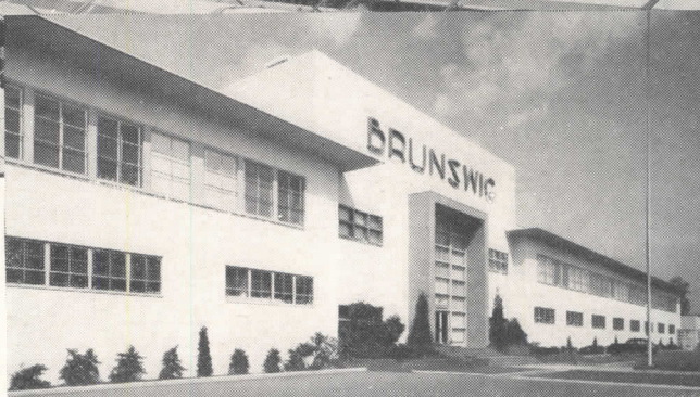
128,000 sq. ft. of 1 9/16" Cemesto provides insulation, interior finish, and great strength with light weight — applied as structural roof deck to the curved roof of Brunswick Drug Company's new plant, Los Angeles, California.
