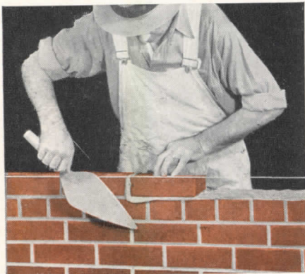
So the mortar will still be soft and plastic when the brick are bedded.
