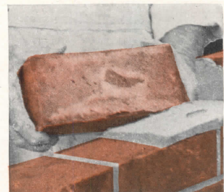
Therefore the mortar did not stick to the top brick. A good bond was not secured.
