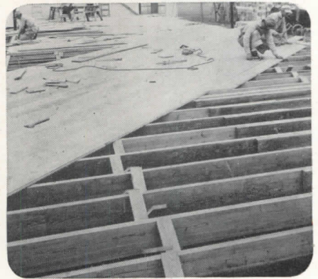
3. Wood used in or near the ground open to attack by termites.
