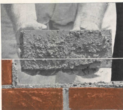
Then the mortar will stick to the brick on top of it as well as to the brick below it.
