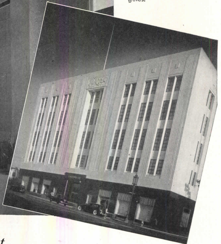
(Below) Marble and polished black granite façade of the store, built by William Simpson Construction Co., Los Angeles.
