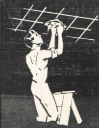
Attach hanger strap to outlet box.
