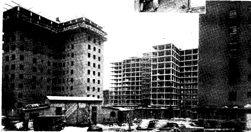
Truscon Diamond Metal Lath Used in Elliot Housing Project, New York City.
