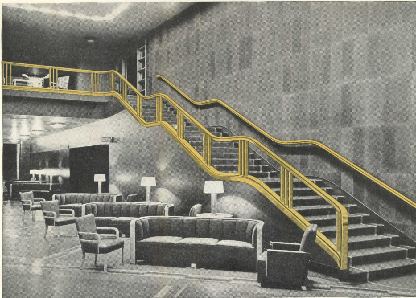
Lobby of The Albany Hotel, Denver, Colorado, Showing railings fabricated from Anaconda Architectural Bronze.
