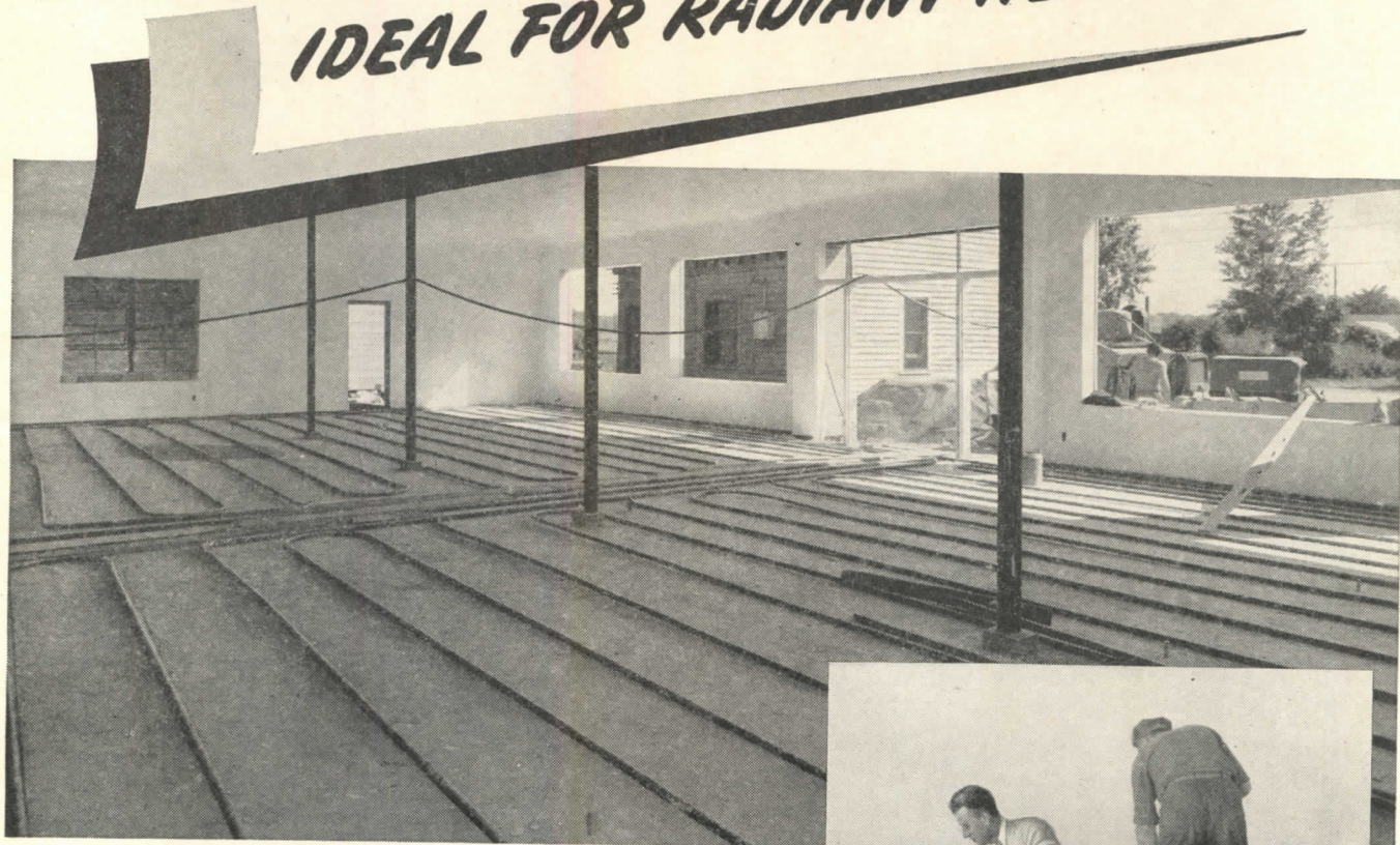
Radiant Heating Coils resting on Zonolite Insulating Concrete
