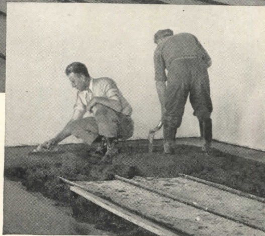
Covering coils with a topping of ordinary concrete
