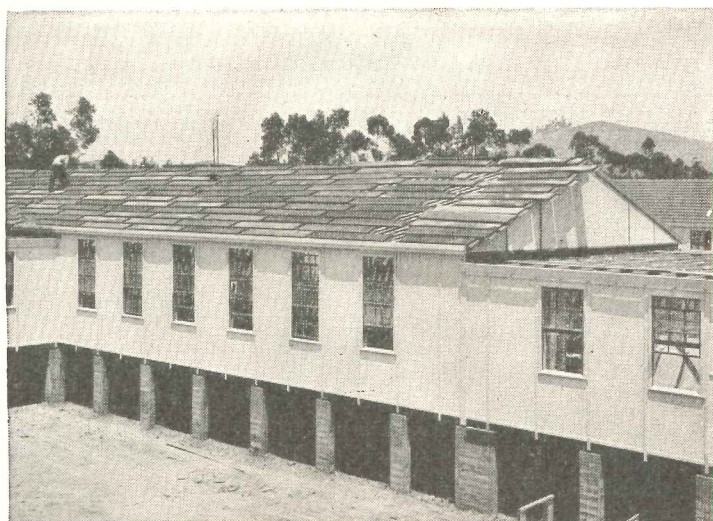
Cemesto walls on one of the sections of the large Naval Hospital at Corona, Calif.
