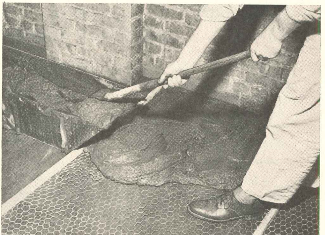
A floor fill consisting of Armstrong's Flormastic, Lumnite cement, and sand is recommended for badly worn or damaged subfloors. When used over wood subfloors, chicken wire should be nailed in place to reinforce the floor fill. Flormastic quickly dries to a hard, smooth finish and can be used as soon as it is dry.
