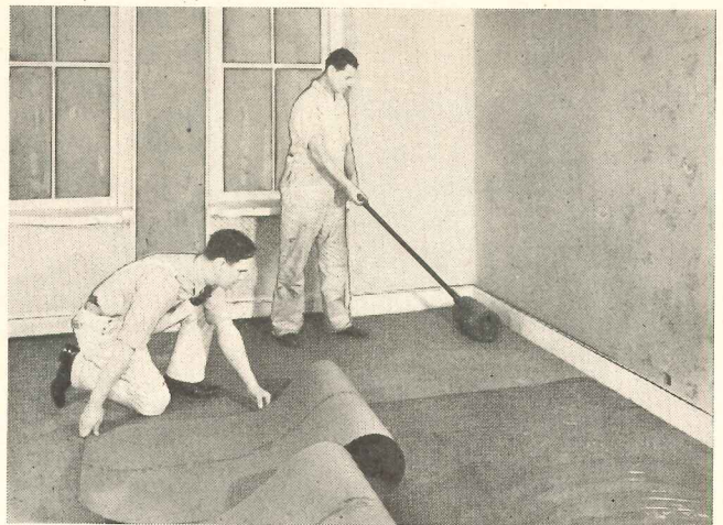
Lining felt should be installed with the strips placed at right angles to the floor boards. It should be cut to fit accurately with a minimum of seams. The felt should be firmly bonded to the adhesive-covered subfloor by rolling out from the center in all directions.
