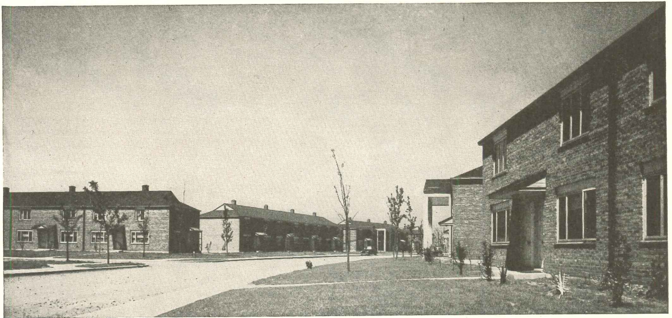
Second unit, Princeton Park Housing Project, Chicago; Holsman & Holsman & Klekamp, architects, Chicago
