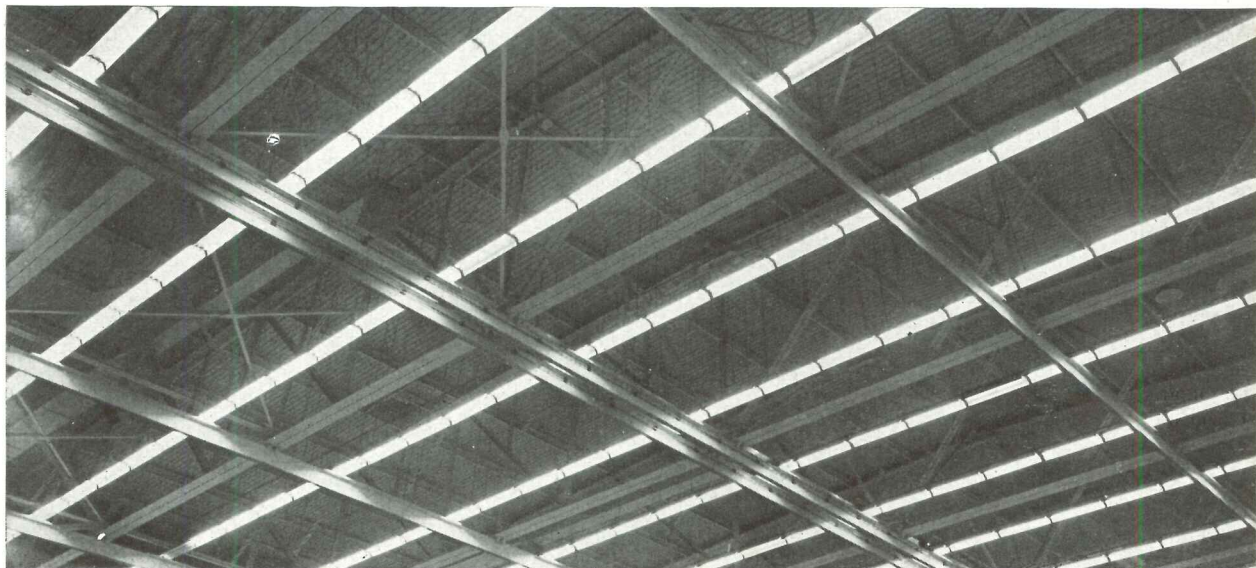
Above, fluorescent lighting in a monitored daylight plant. In the near future, fluorescent will have to compete with cold cathode. Below, lights in a complete "blackout" plant, giving full control and low maintenance but raising questions of effect
