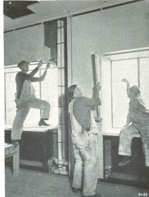
Installing pier and window embrasure. Deep window recesses and inset interior wall leave plenty of room behind for heat and utility pipes
