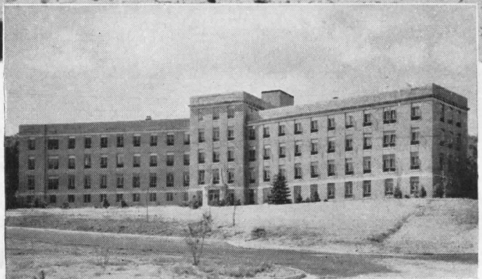
The Mt. Washington Sanitarium, Eau Claire, Wisconsin. Equipped with the new Ceco Intermediate Casement.
