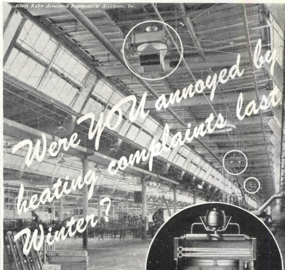
(Above) Installation of 03 WING Revolving Unit Heaters in Plant of Automotive Appliance Manufacturer
