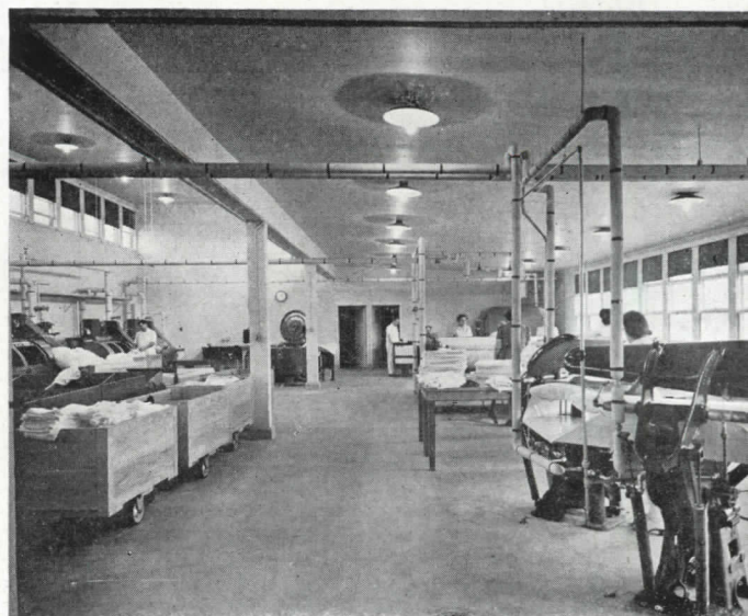
Right center: the nursery is equipped with cubicles made of shatter proof glass and plywood. At the bottom is a general view of the laundry. Note large windows near the ironers, and monitor type over the washing machine area
