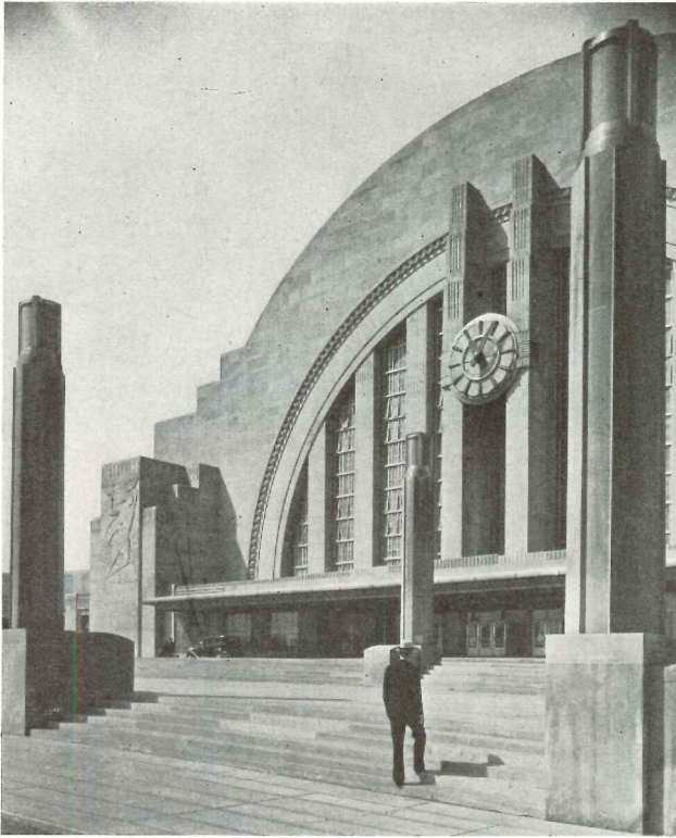
Union Terminal, Cincinnati. Fellheimer and Wagner, Architects, the famous railroad station built in the early thirties. A feature is the excellent handling of buses and rapid transit. The front is toward the city; tracks to the rear are parallel to its face; an opportunity for a monumental frontal approach
