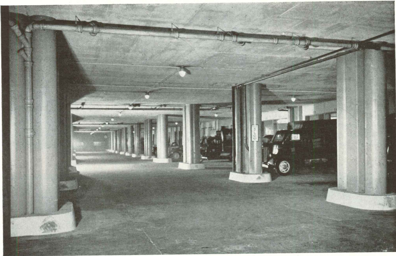
Tail-gate parking at sub-track level of station
