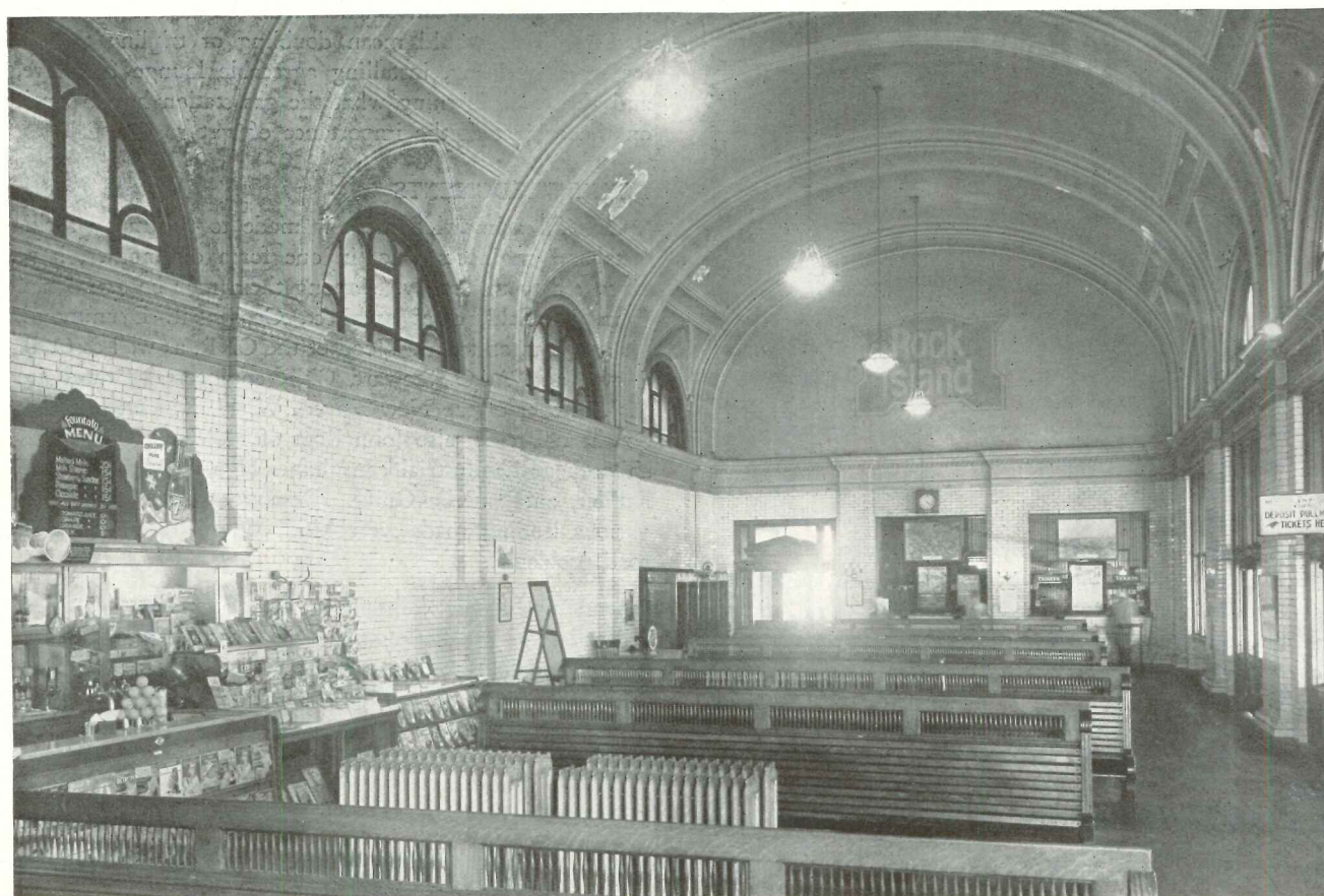
This modernization of the Rock Island station at Des Moines is typical of the kind of change that can be made in countless other railroad stations. The ticket window that shows at the end of the lower picture was removed and an open counter placed at the center of the long wall, right, next to train platforms. The sloppy newsstand, front below, was removed. Instead, a newsstand was placed in one angle where it may be seen in the view above, balanced by a lunch counter in the opposite angle, both so designed as to remain within proper confines. The long benches, which so manifestly block progress through the station, were replaced by lounge furniture. Fluorescent cove lighting replaced the hung lights. Although the tile wall previously in use was easy to maintain, it was covered by walnut veneer, far less glaring for passengers to look at. The glass block panels introduce light from the street side, where it was decided to exclude the view. Work was done under direction of D. A. Ruhl, chief engineer; Otto Kuhler, consultant
