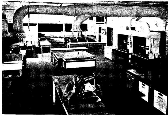
Kitchen is ventilated by exhaust ducts and fans in gable ends
