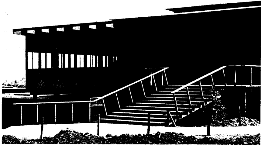
Hillside Dormitories, Vallejo, Calif. Right, entrance to coffee shop; below, dining room. Vernon DeMars, FS.1 Architect; Norman Fletcher, Associate
