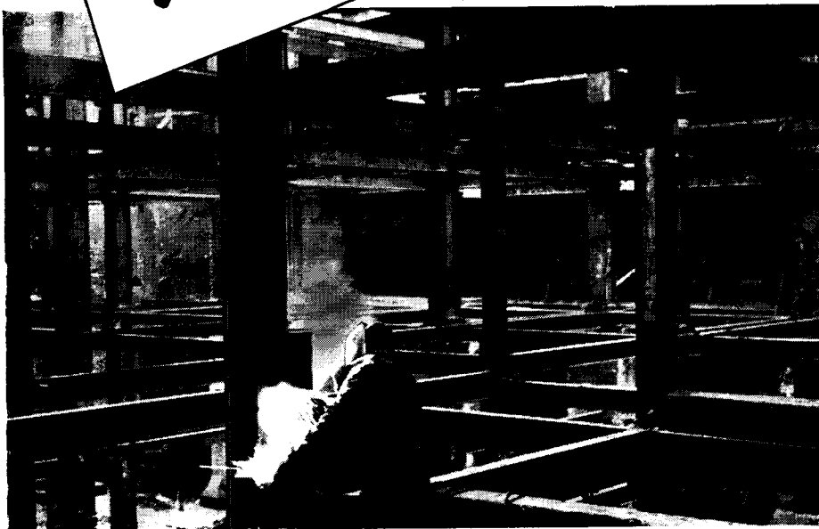
Right: Nurses' Home, Jersey City Medical Center. All welded construction—23 stories high—2200 tons of structural steel.
