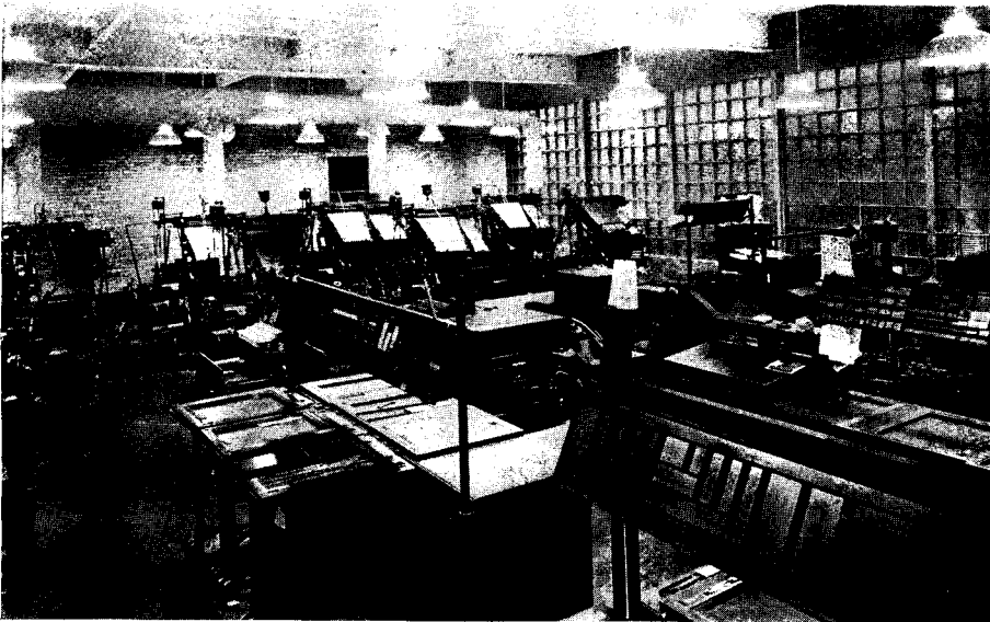
In the composing room, vitreous brick walls, glass block window lights, strong overhead light, give every inducement to keep things clean. All shop floors are of wood block, laid on end
