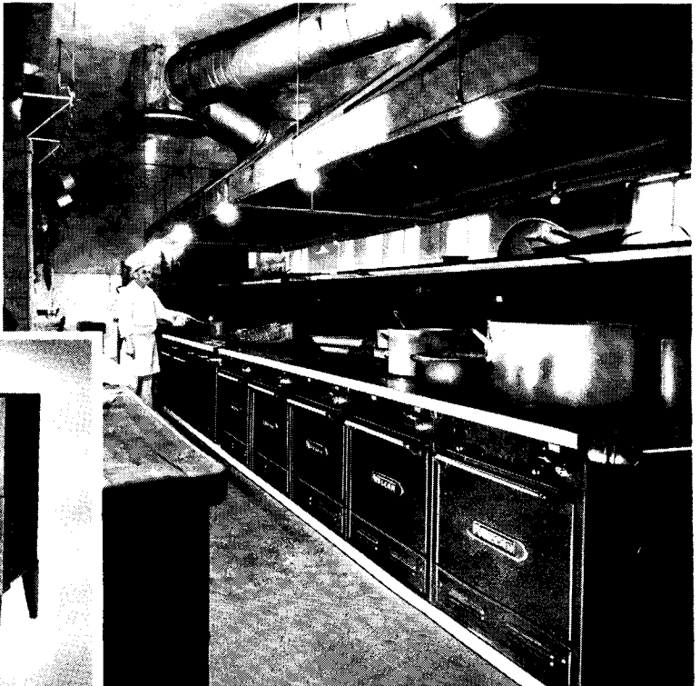
SPECIAL SERVICE REQUIREMENTS are handled by this arrangement of Vulcan units. Ranges are grouped to give cooks unobstructed facilities. Note alternating open and closed top ranges at right of battery—bank of fryers connected to left of ranges with broiler following.
