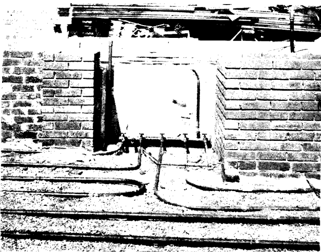
Individual valves for balancing the system are conveniently located in a typical return header installation
