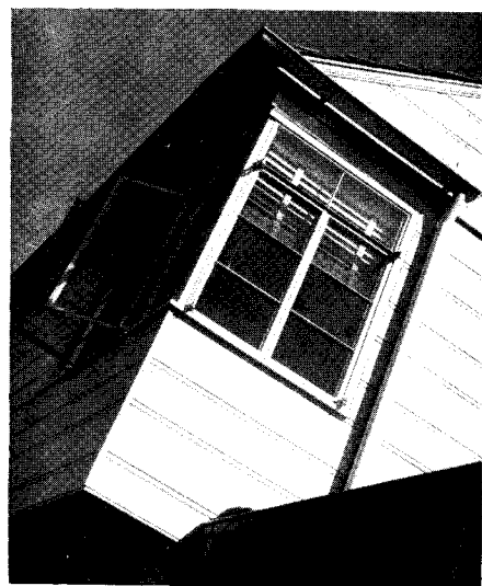
Gutters are carried around the corner, to keep downspouts off the front
