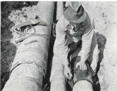
Installing connector band. All necessary accessories are prefabricated and shipped with order.
