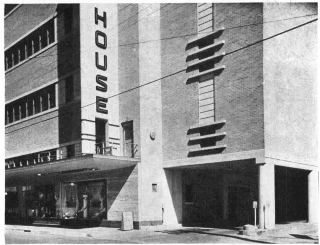
Vehicle driveway to parking lot at rear
