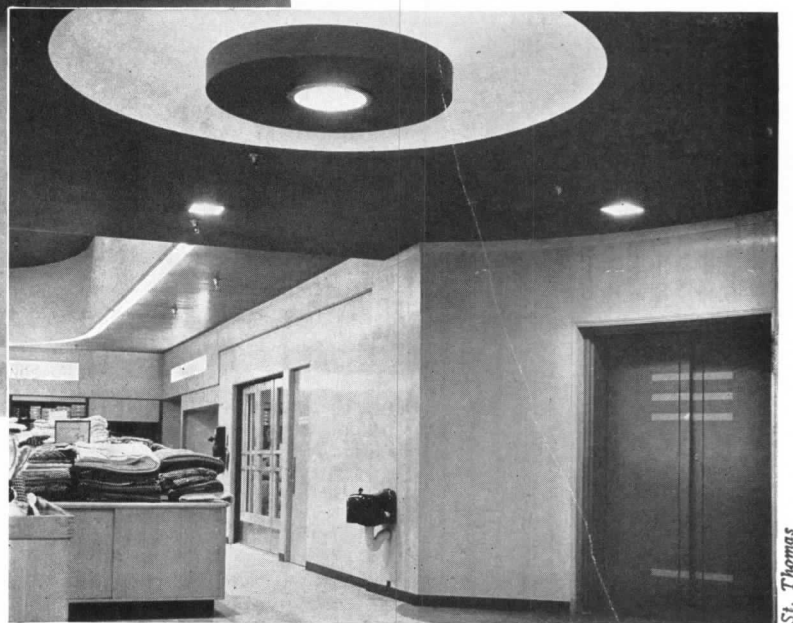
View (above) from first-floor elevator landing to main entrance on Orleans St. Floor here is terrazzo; store equipment fixtures are of bleached pin oak and prima vera. A complete sprinkler system was installed; pipes are concealed
