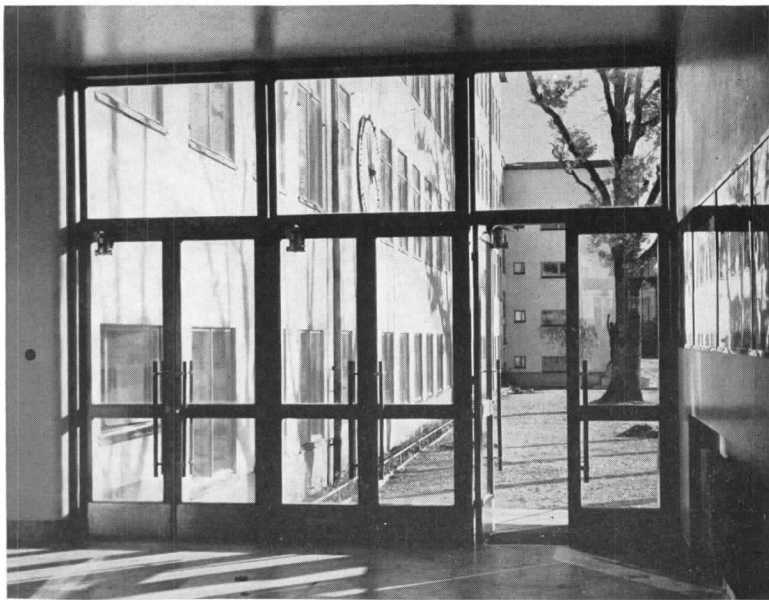
Openings are glazed to the utmost for light and sense of spaciousness. Entrance doors, BROMMA SCHOOL, Stockholm. At the right, simple pre-fabricated concrete risers and treads are laid on reinforced concrete stair beams in the ERIKSDAL SCHOOL
