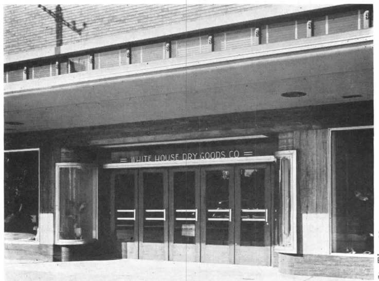
Main entrance on Orleans street
