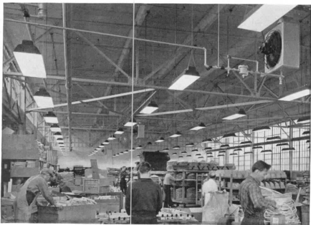
While many modern installations use fluorescent lamps in continuous rows, with this type of lamp it is possible to achieve good even lighting with fewer fixtures placed at fairly low height
