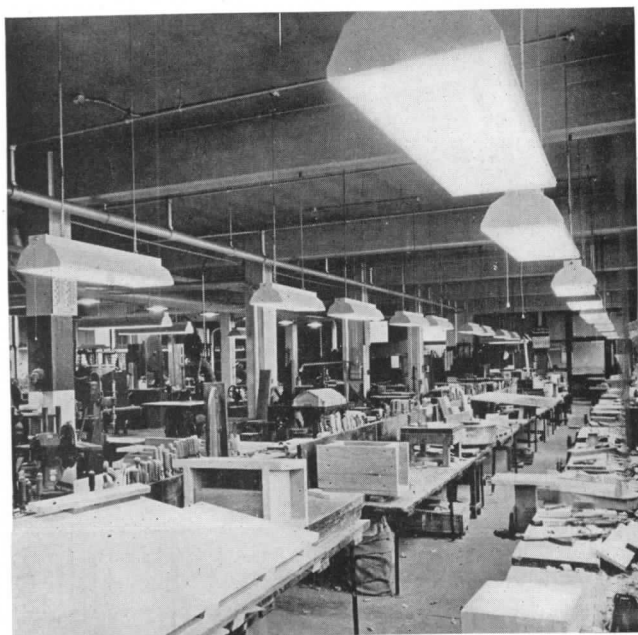
To deliver 75 foot-candles at the bench level of this pattern department of a large Eastern concern, fluorescent fixtures were placed just 7 ft. above the floor, on 6 ft. by 9 ft. spacings
