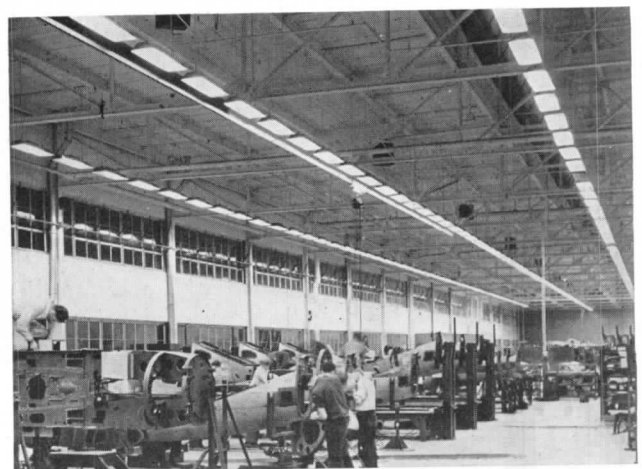
Fluorescent lamps in rows of individual fixtures give uniform lighting for the manufacture of fighter planes, with high intensity light and a minimum of shadows at the level of the work
