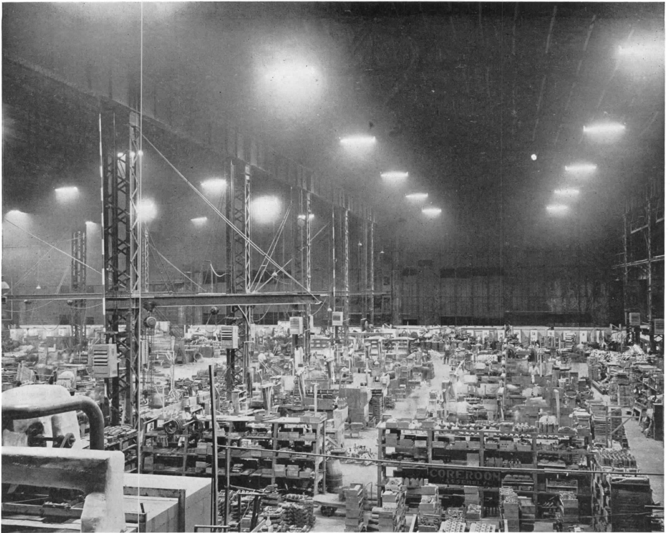
An area of 22,000 sq. ft. is lighted by 220-400 watt mercury lamps mounted at a height of 32 ft. They provide about 60 foot-candles of illumination for the critical visual task performed
