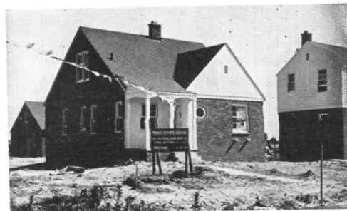
Now becoming rare in defense housing is brick veneer construction. This group of
