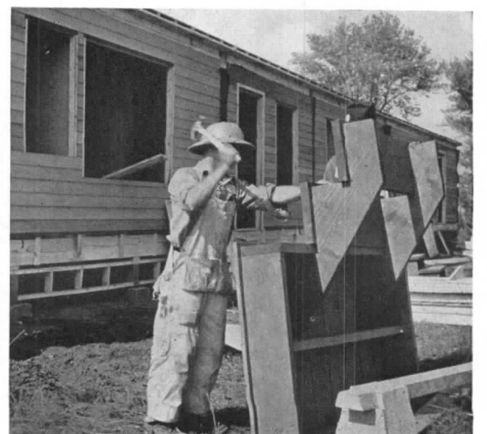
each other at the peak. Shingles go over plywood sheathing. 3. Sub-assembly at the site produces porch steps, underpinning, front door hoods
