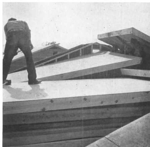
1. Ceiling panels and roof sections are raised by means of a greased skid. 2. Roof pitch is achieved without trusses by propping two sections against
