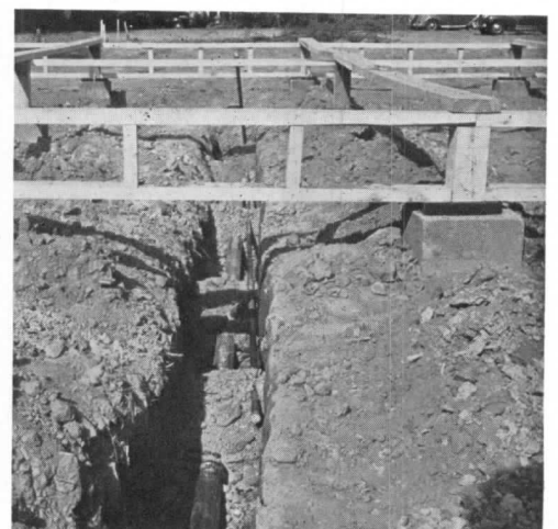
brought from the factory to the individual lots. 3. Soil stacks and piping are already laid and the house underpinning is in place to receive them
