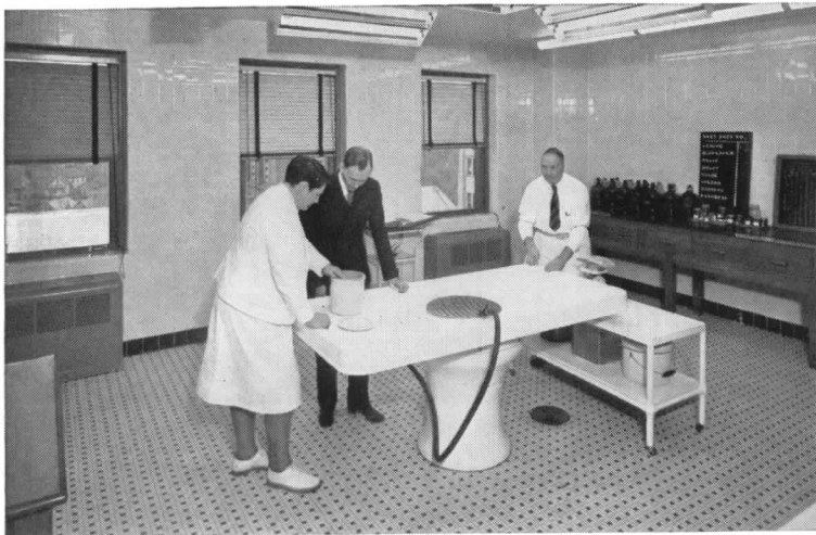
POST-MORTEM s are conducted with very latest type equipment in the post-mortem room in the new eight-story addition at St. Francis Hospital. Conditioned air is provided by the revolutionary new Carrier Conduit Weathermaster System. No chance for circulation of disease germs and objectionable odors from one room to another.
