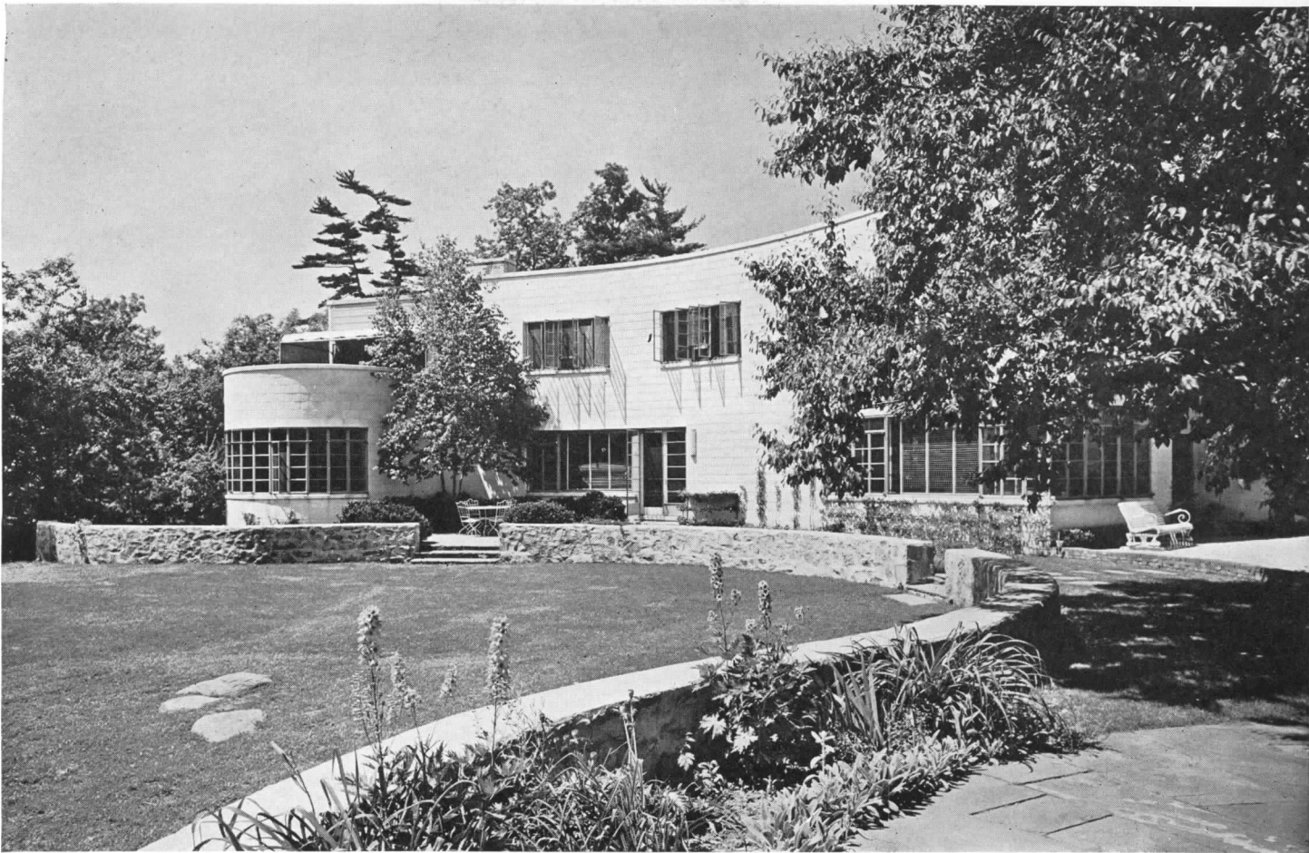
South facade and terrace as viewed from the pool end of the terrace wall
