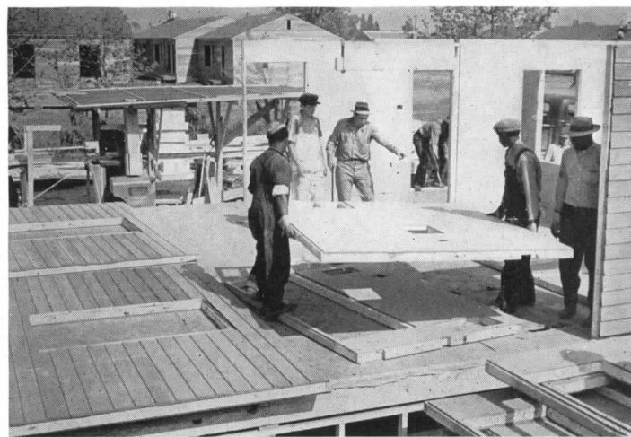
D 1. Floor panels are raised on the underpinning. As soon as floors are laid, heavy building paper is laid over them to protect them during re-
