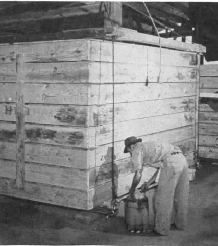
1. Panels, surfaced on the inside with insulating board, are stacked, ready for transportation to the site. 2. Hoisted on trucks, they are
