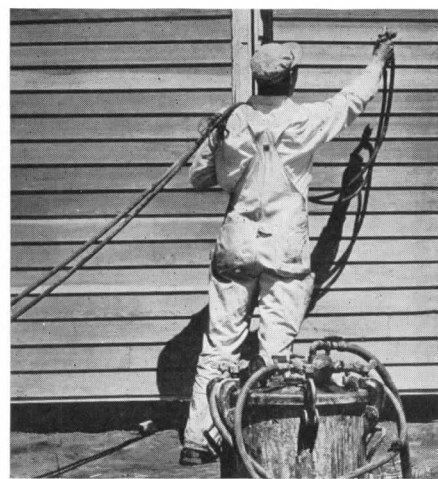
F 1. A row of houses, nearing completion; the siding is redwood. 2. A creosote mixture is sprayed on exterior walls with a spray gun and com-
