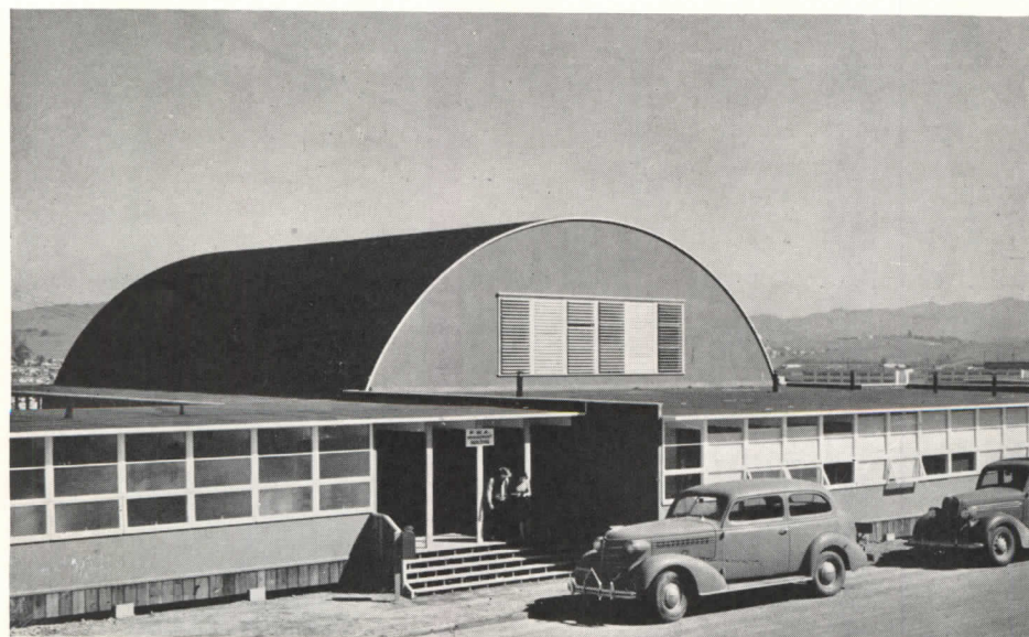
EXTERIOR WALLS are painted; the roof is mineral-surfaced composition roofing rolls
