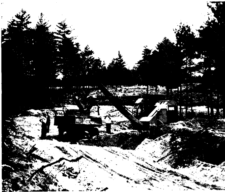
MARCH, 1940: Work on new site under way
