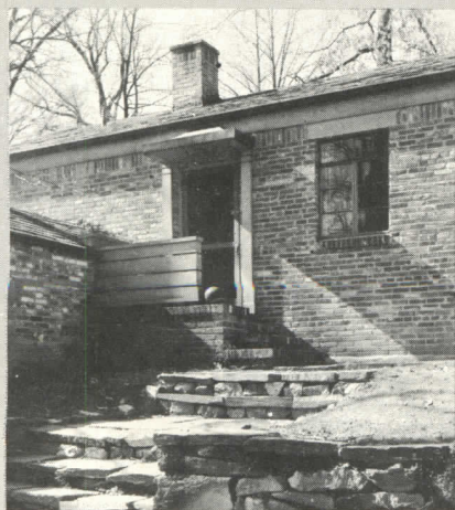
FRONT DOOR (Garage at left)
