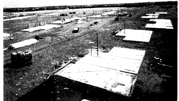
CONCRETE SLAB FLOORS and foundations
