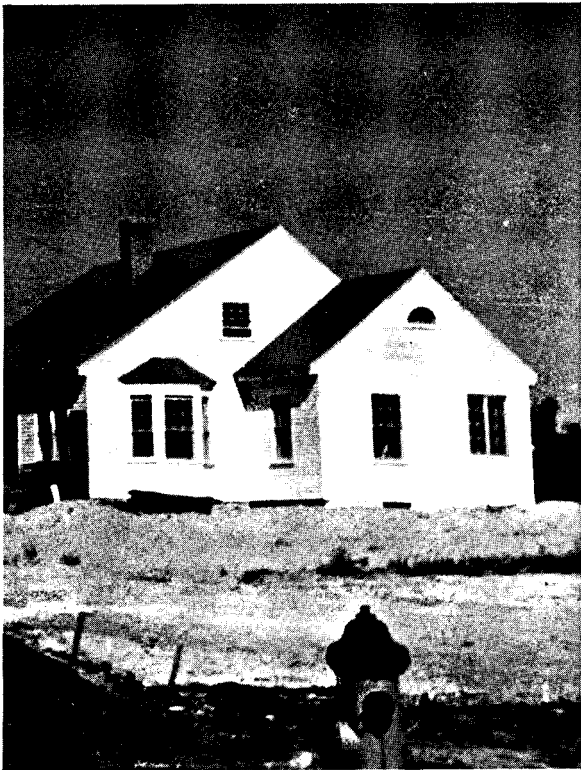
Above, a residential street in the new village; at left, similar view in the old
