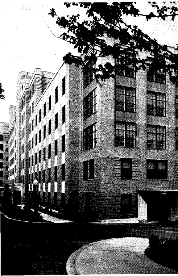
Photos, left to right: exterior; main entrance; clinic entrance; lobby, Unit 1; clinic lobby, Unit 2. Structure has reinforced concrete skeleton, brick walls shaded progressively lighter from base to coping, limestone trim. Color is extensively used in operating rooms, public and private bed spaces. All possible means of noise control are employed; sources are eliminated or acoustically treated; installation of sound-deadening material is called largest in any privately financed hospital. Signal system operates lights instead of loud speakers or bells
