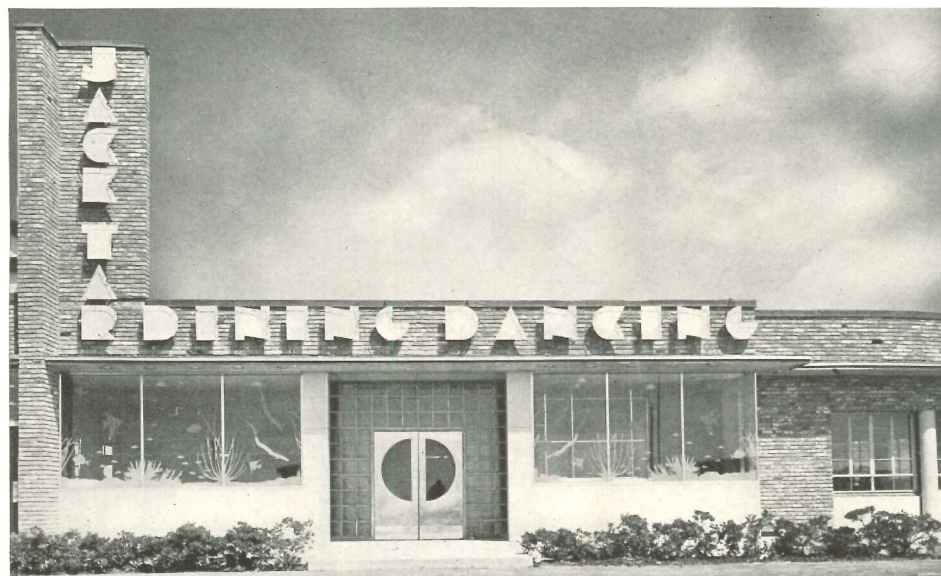
Restaurant's shape (see plan) and decoration are suggestive of a ship's deck.
