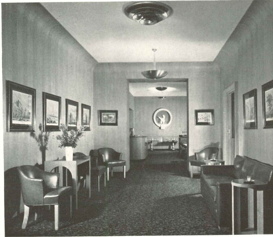
No. 1: From a station entrance, the door leads into No. 2: the carpeted foyer. Walls, white-oak veneer on flexible backing
