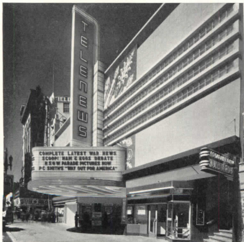
THREE VOTES: Telenews Movie Theater for which Albert F. Roller was architect.
