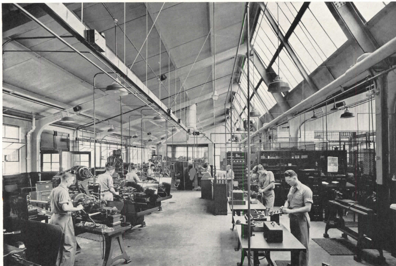
North-light monitors, continuous wall glazing, and structural steel design provide extraordinary daylight conditions.
