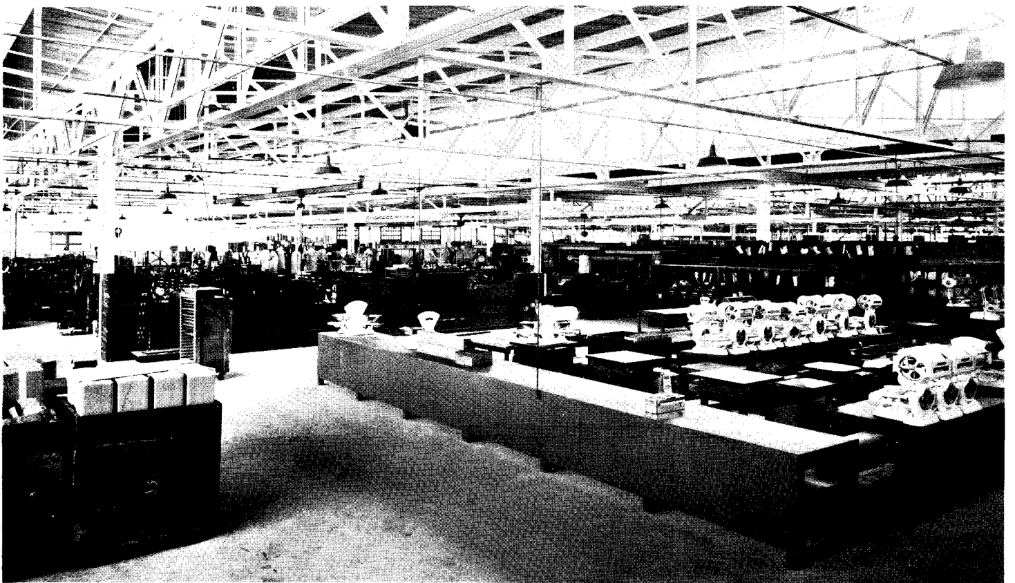
Inspection area: good light is assured by monitor design and by movable direct lighting fixtures fed from trolley ducts.
