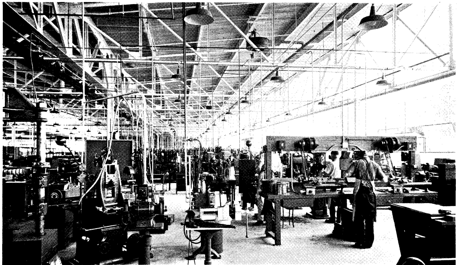
General manufacturing area: note new projection-type unit heaters and bus-duct power distribution.
