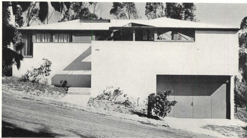
Top: the outdoor living deck. At right, in order: general view of the front; the south- ern end; the rear of the house.
