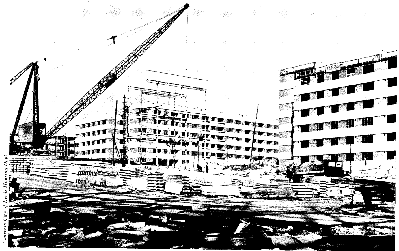
Concrete units ready to be raised to position; the units are supported on vertical posts notched to receive them.
