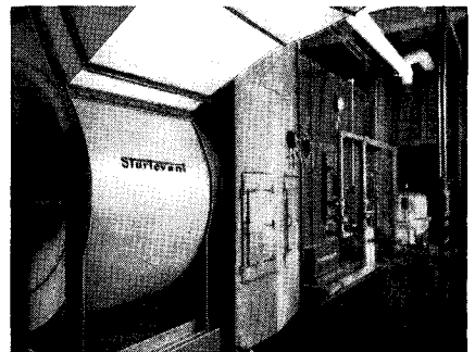
Photos show two of the Sturtevant Silentvane Fans and one of the Sturtevant Air Washers installed in Southern New England Telephone Building, New Haven.
