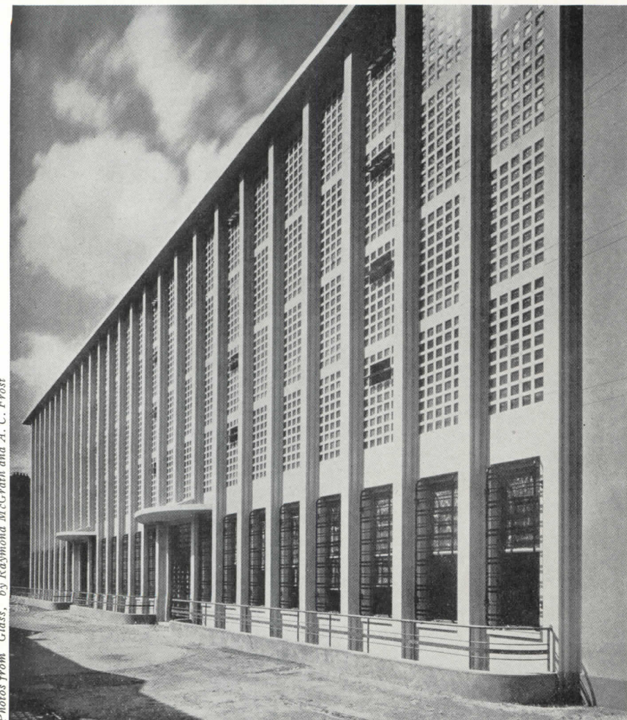
Fig. 7. Using a glass block similar to American ones, architect Roux-Spitz has developed a prefabricated wall unit of greatly increased efficiency in this library at Versailles, France. Here load-bearing properties of glass are in full use.
