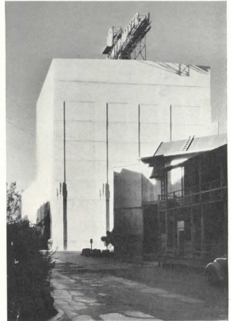
An old-type sound stage; the walls of the structure are solid concrete and insulation is proportional to wall thickness.
