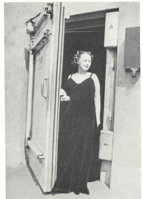
Pedestrian door of one of the new sound stages. No single door can provide insulation value equal to that of stage walls: a pair of doors, with a 5-ft. air space between them, is provided.
